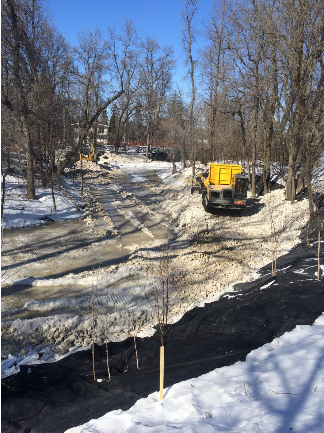
Photo 4 - Rockfill toe berm placement at 3144 Henderson Highway.
