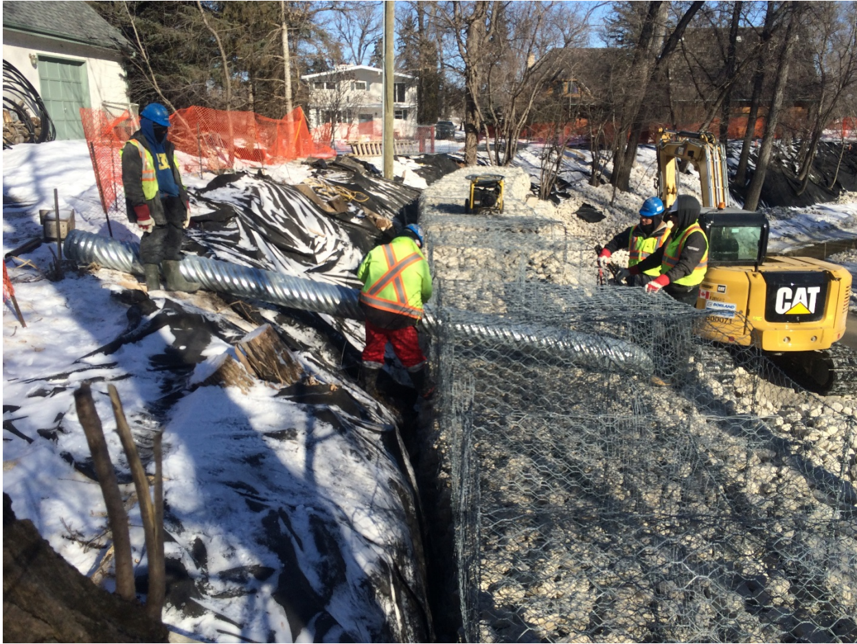
Photo 5 - Installing culvert through gabion baskets at 1030 Highland Park Drive.
