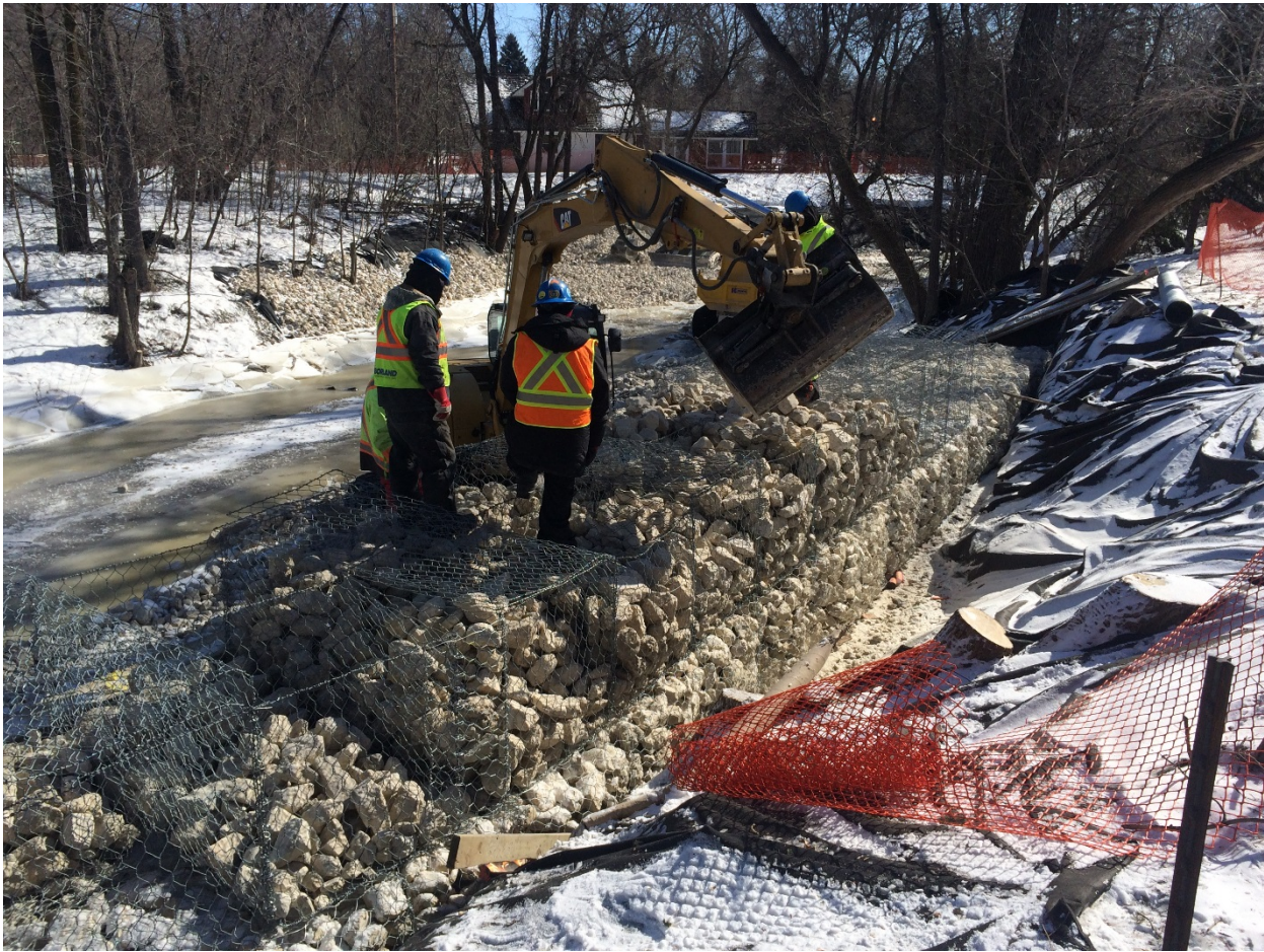
Photo 3 - Filling gabion baskets at 1030 Highland Park Drive.
