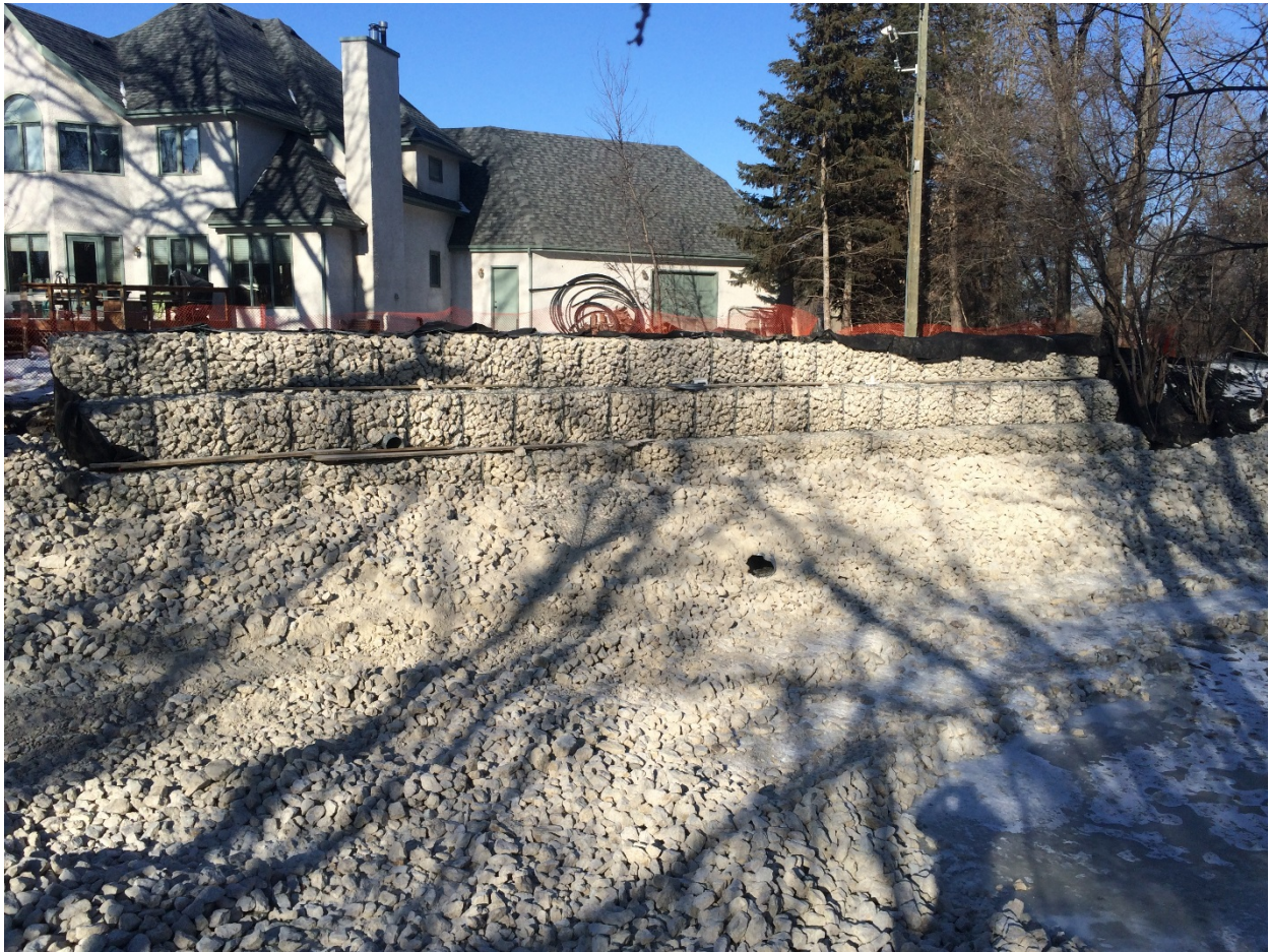
Photo 6 - Completed gabion baskets at 1030 Highland Park Drive.
