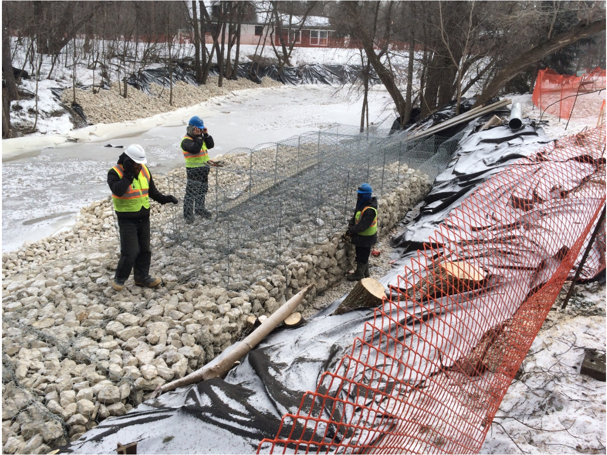
Photo 2 - Installing gabion baskets at 1030 Highland Park Drive.
