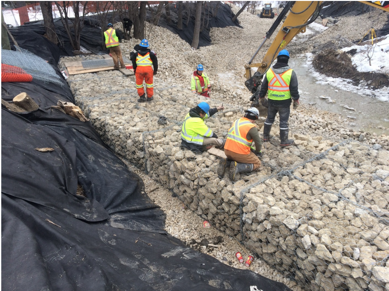
Photo 1 - Filling gabion baskets at 1030 Highland Park Drive.
