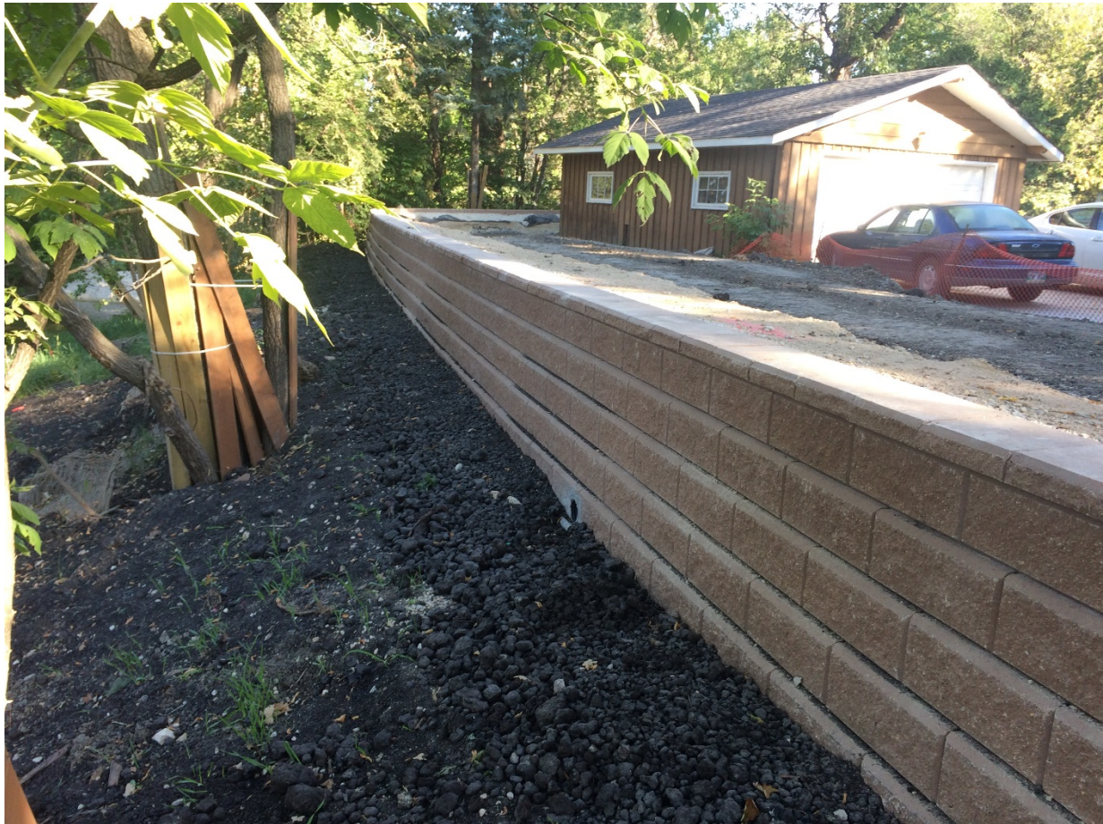
Photo 6 - Capstones placed on creek side segmental block wall at 3144 Henderson Highway.
