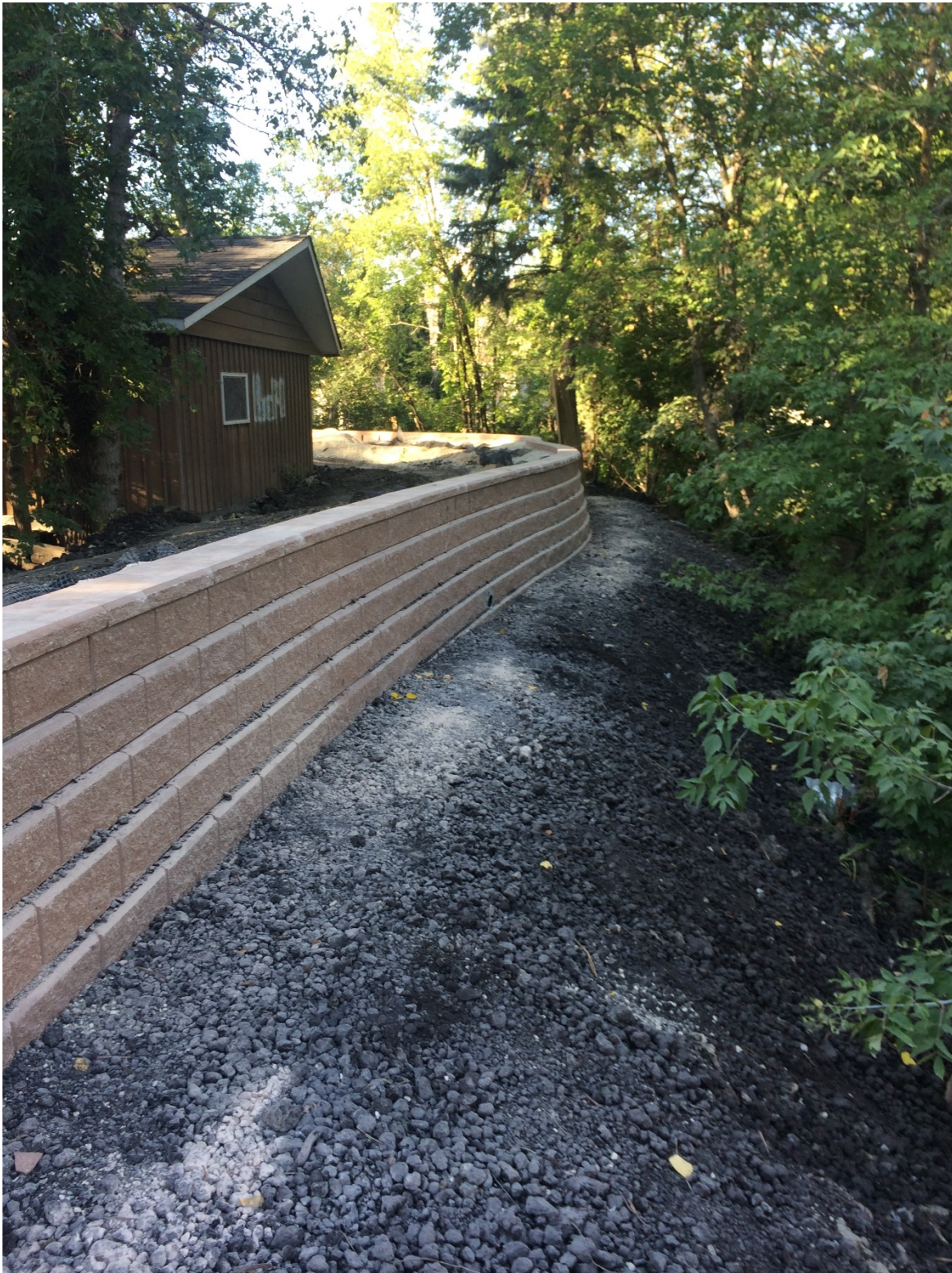
Photo 7 - Capstones placed on creek side segmental block wall at 3144 Henderson Highway.
