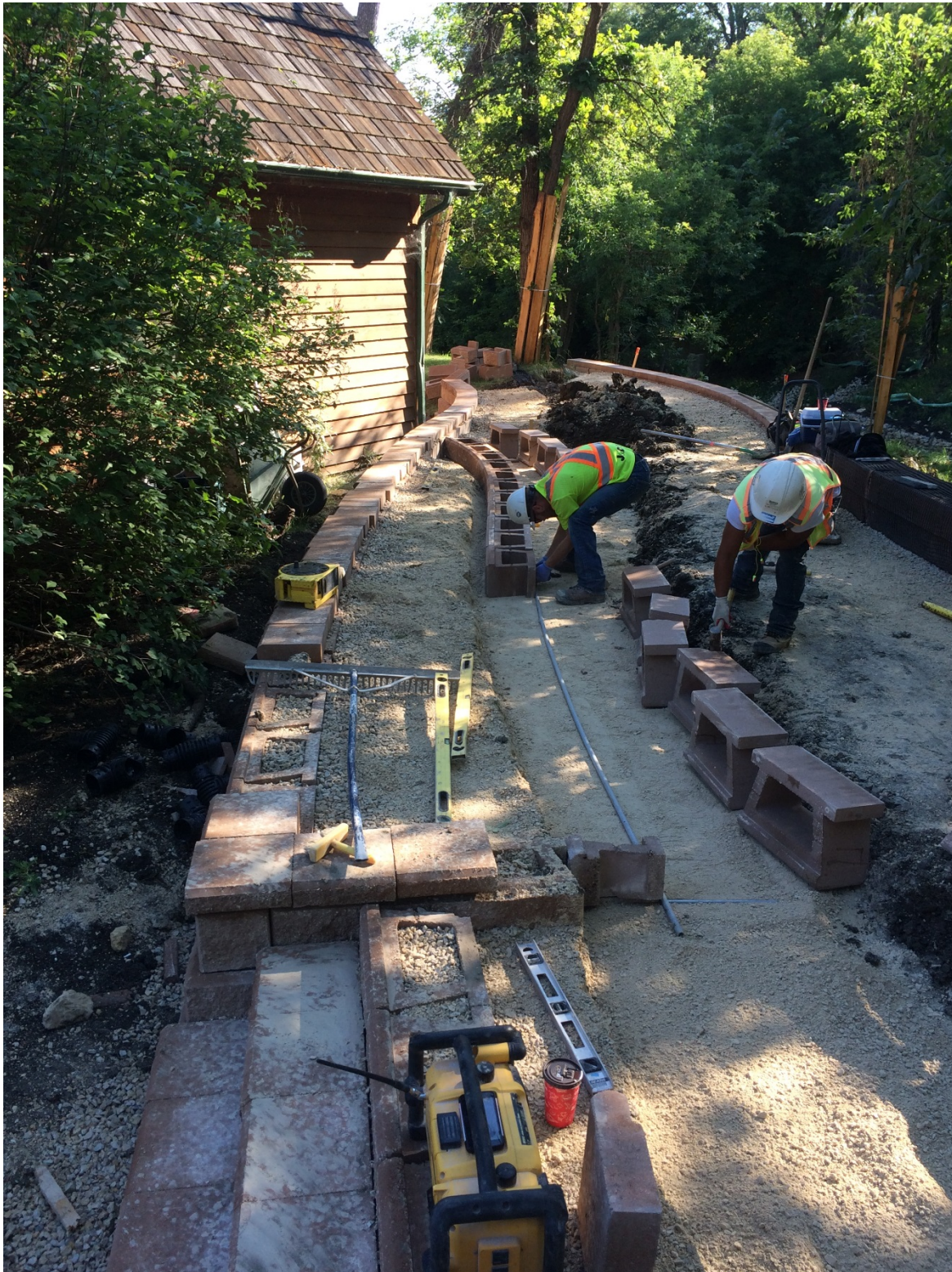
Photo 4 - Placement of terraced segmental block wall at 1040 Highland Park Drive.
