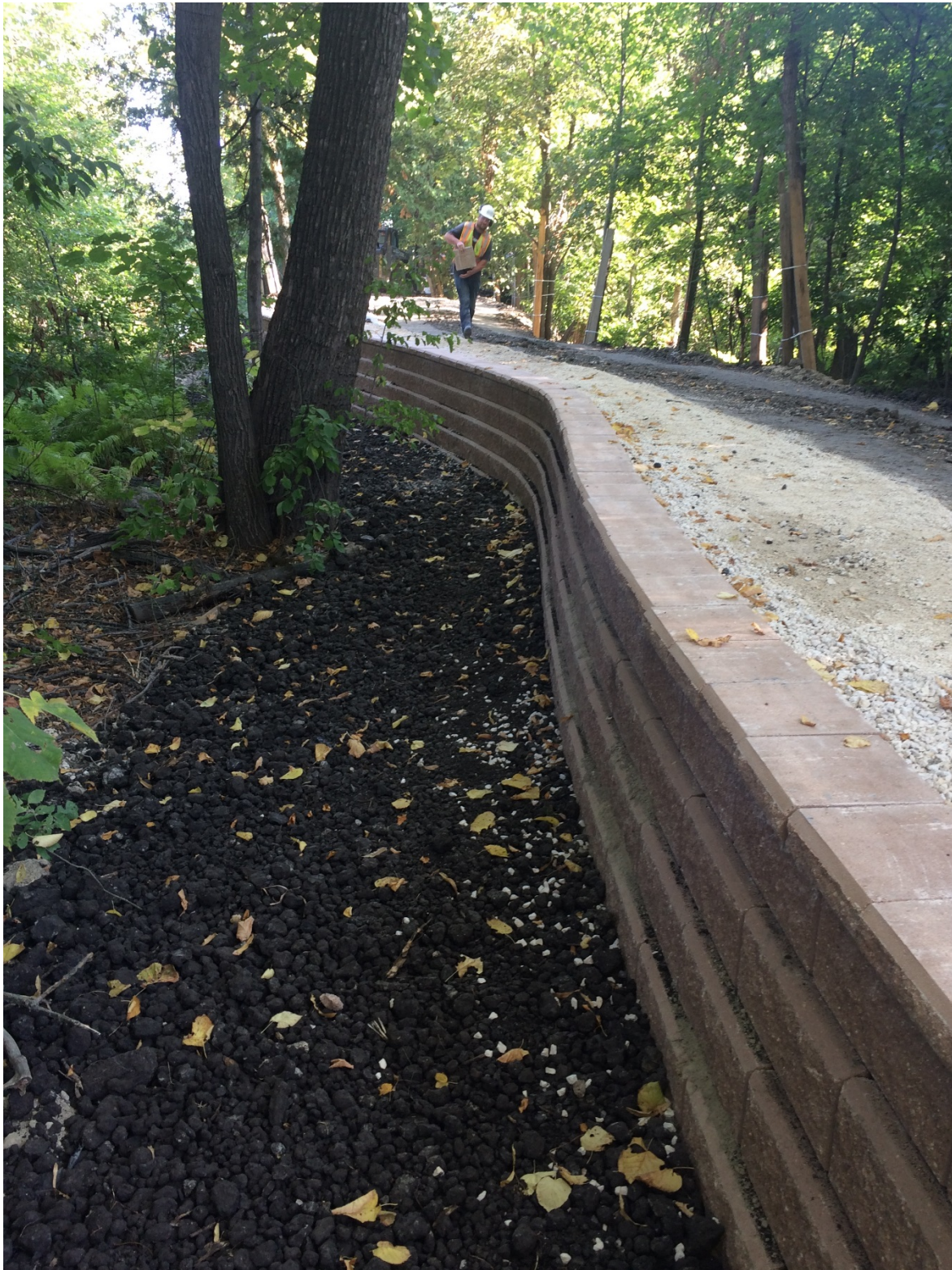
Photo 8 - Capstones placed on creek side segmental block wall at 3154 Henderson Highway.
