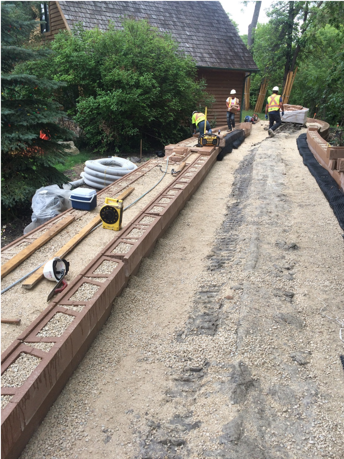
Photo 5 - Placement of terraced segmental block wall at 1040 Highland Park Drive.
