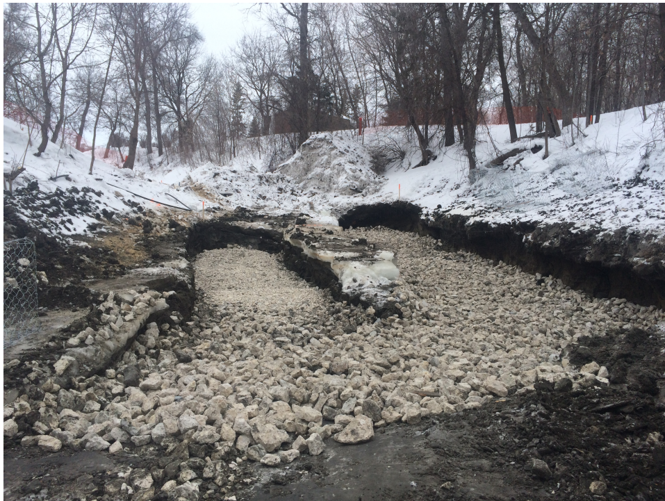
Photo 5 - Shear key rockfill placement at 1040 Highland Park Drive and 3154 Henderson Highway.
