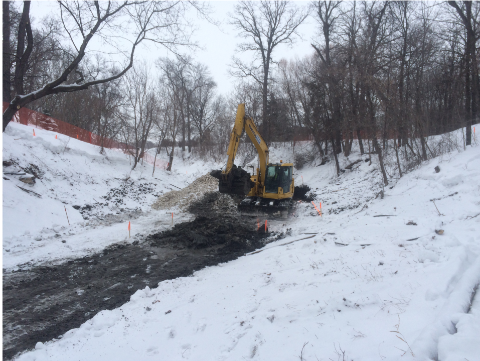
Photo 4 - Shear key excavation at 1040 Highland Park Drive and 3154 Henderson Highway.
