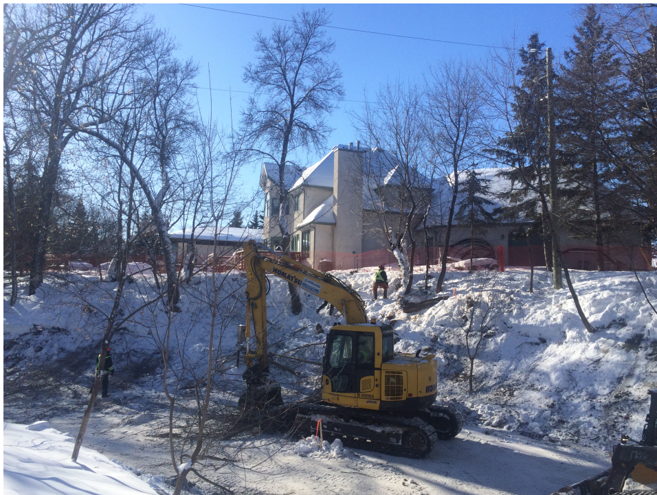
Photo 1 - Tree clearing at 1030 Highland Park Drive.
