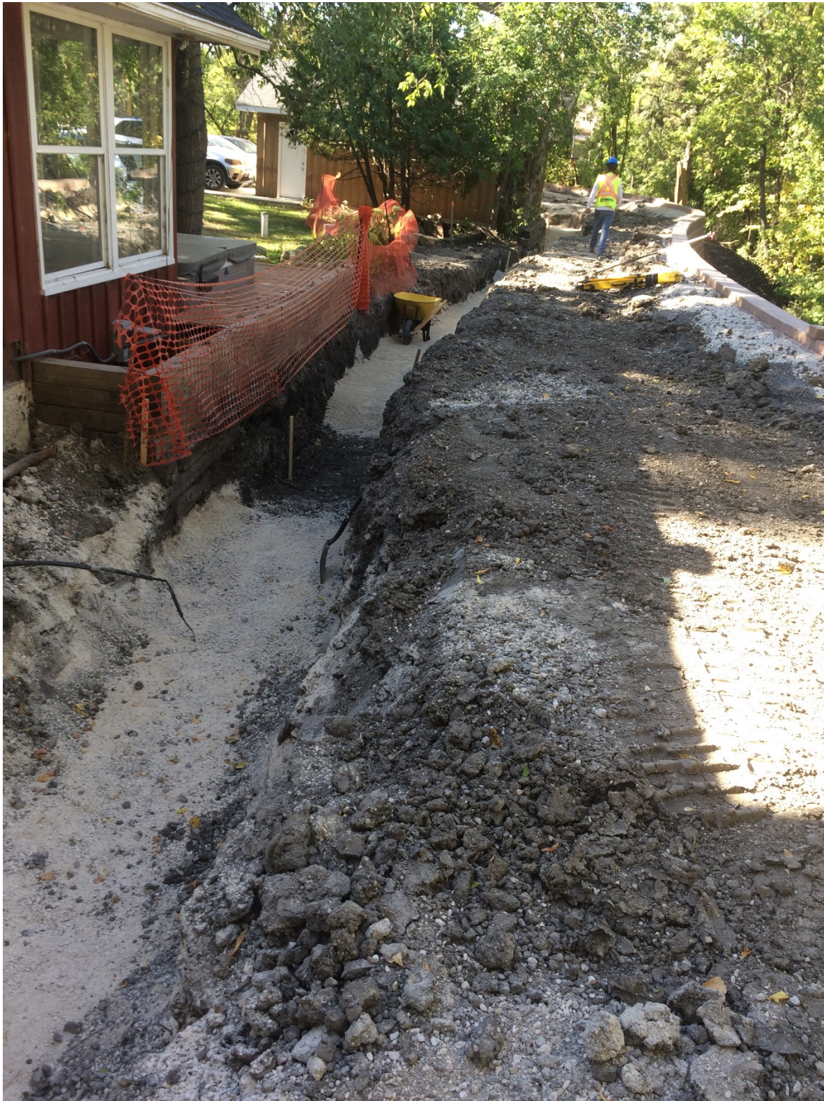
Photo 3 - Foundation for house side segmental block wall at 3144 Henderson Highway.
