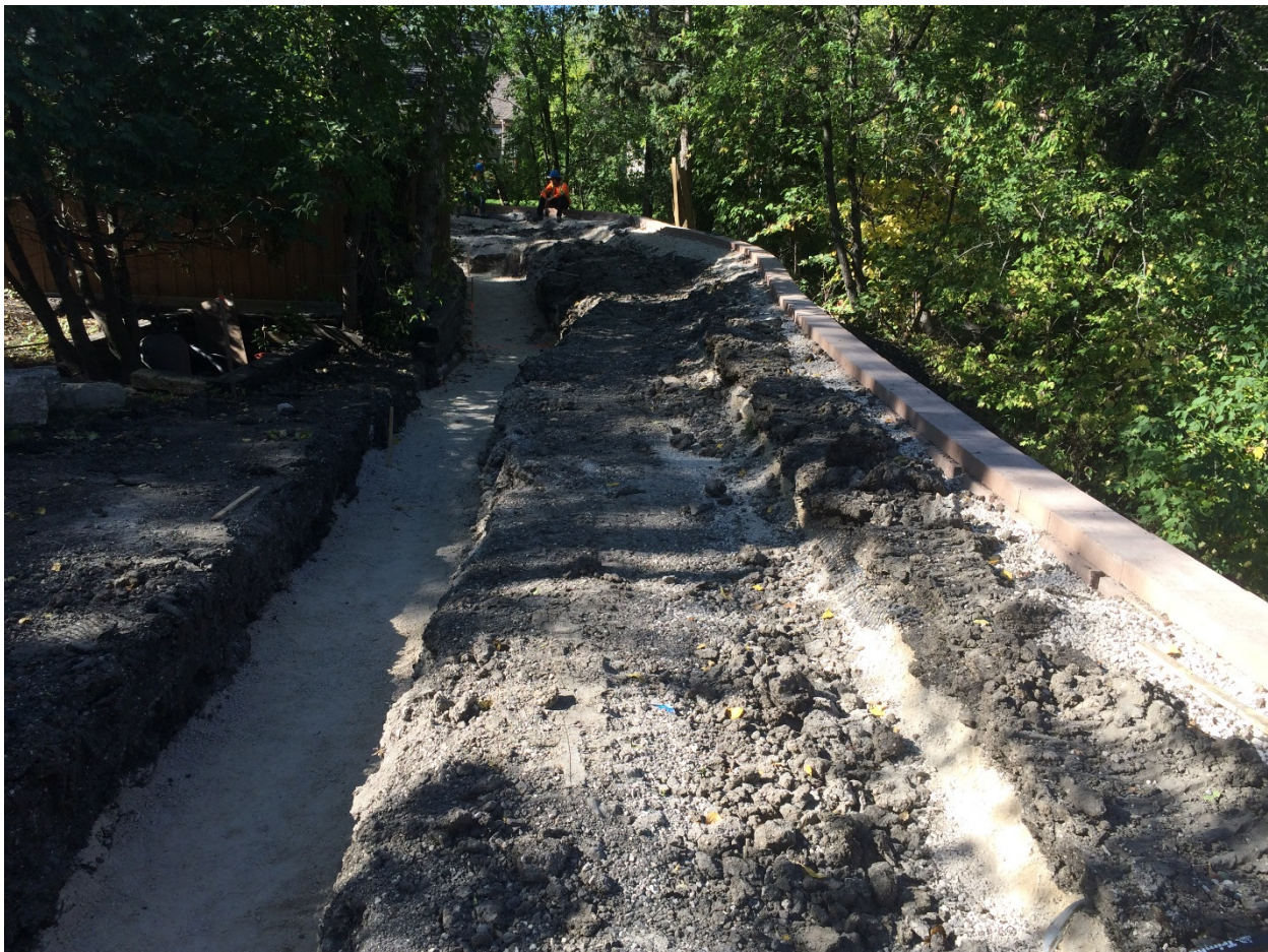
Photo 1 - Foundation for house side segmental block wall at 3144 Henderson Highway.
