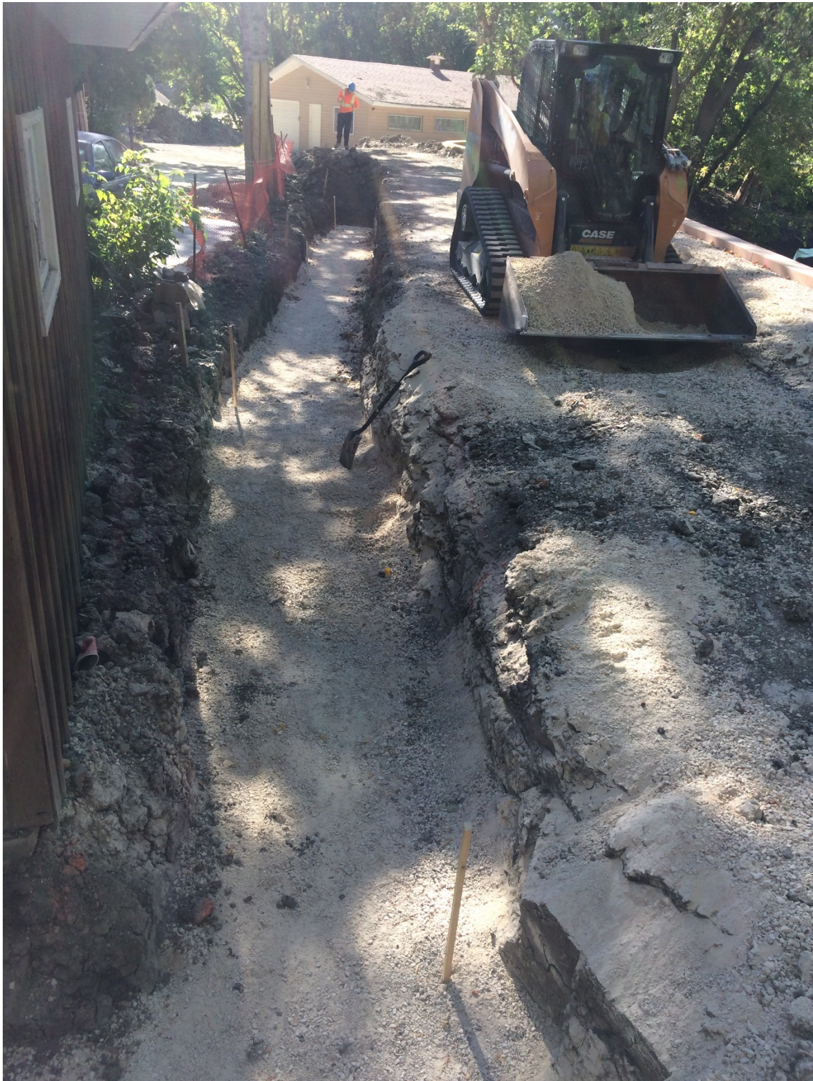
Photo 2 - Foundation for house side segmental block wall at 3144 Henderson Highway.
