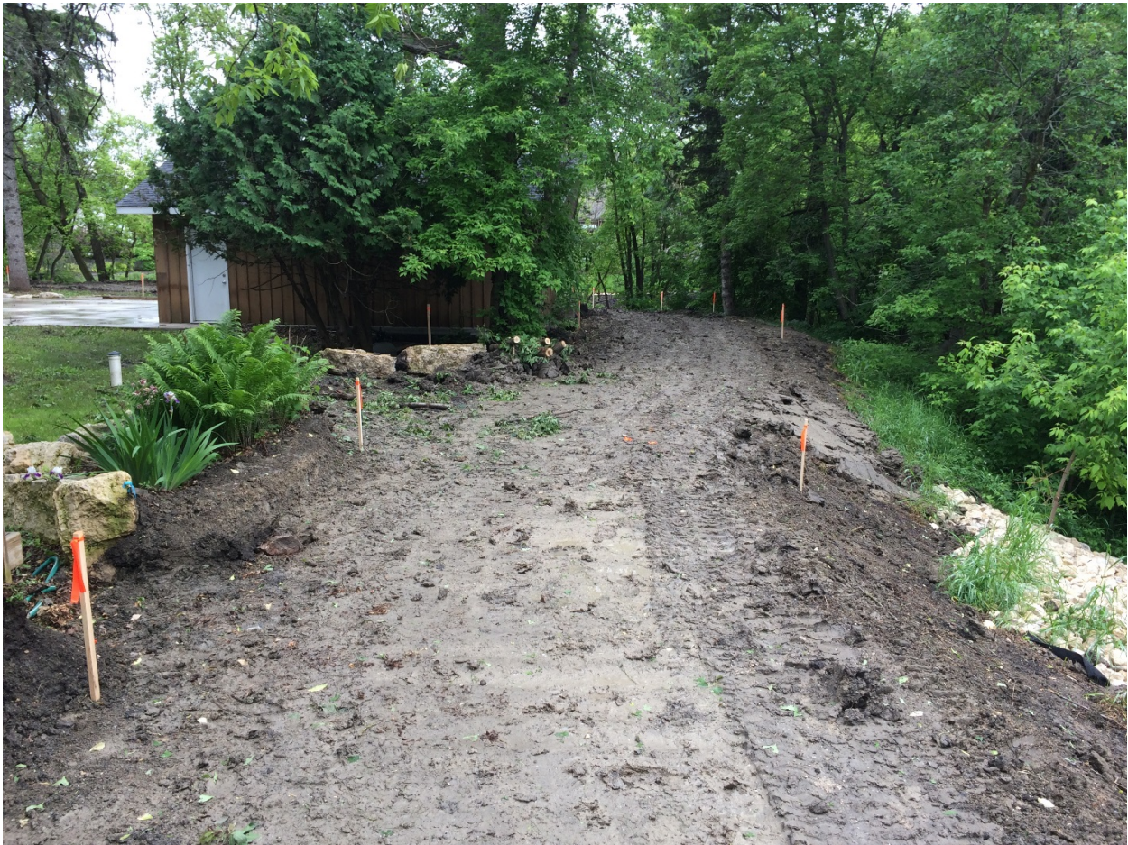
Photo 7 - Existing dike removal at 3144 Henderson Highway.
