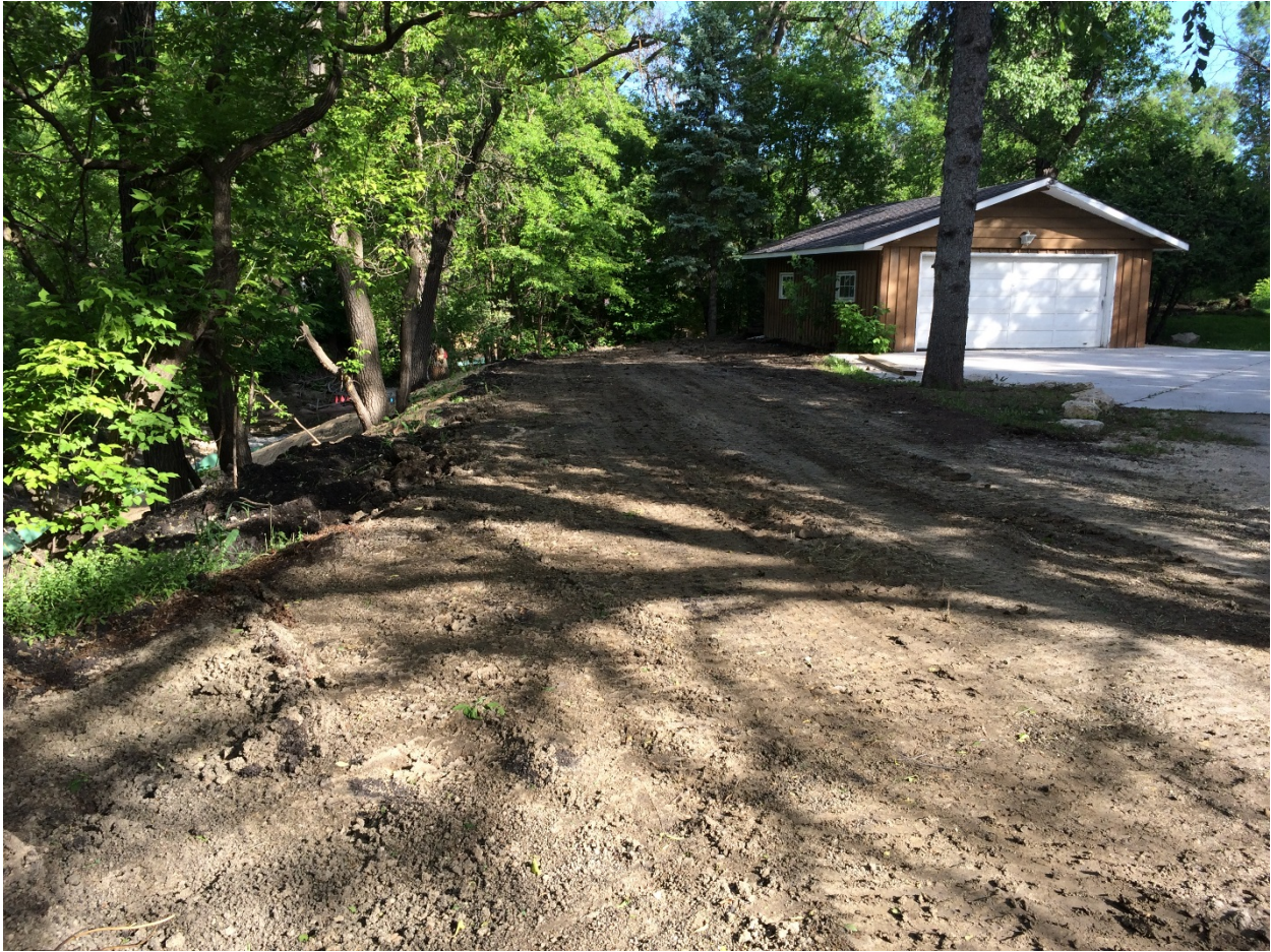
Photo 6 - Existing dike removal at 3144 Henderson Highway.
