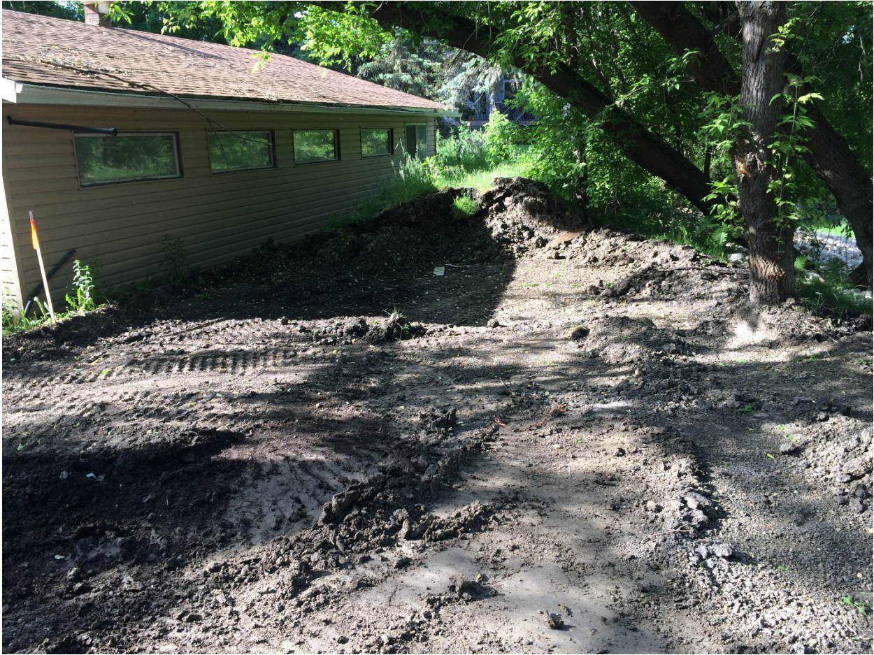
Photo 5 - Existing dike removal at 3144 Henderson Highway.
