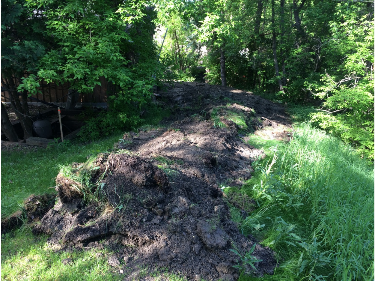
Photo 4 - Removal of organics from the existing dike at 3144 Henderson Highway.
