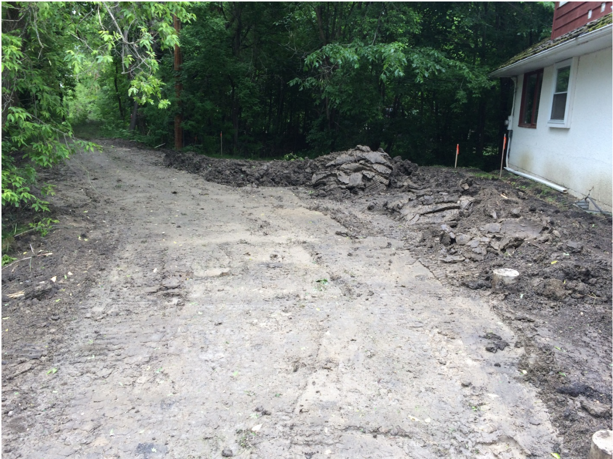
Photo 8 - Existing dike removal at 3144 Henderson Highway.
