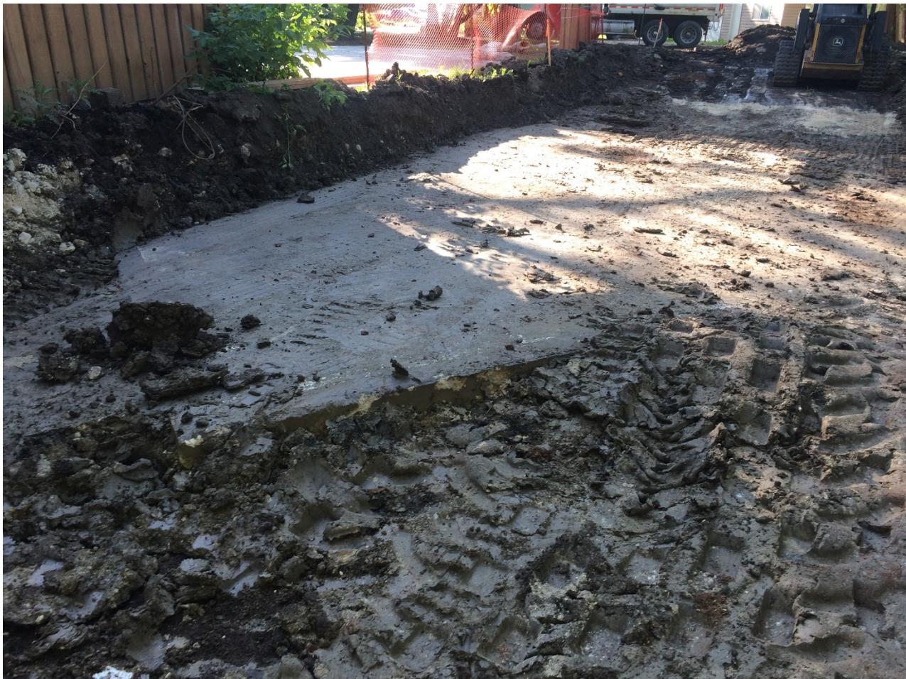
Photo 1 - Concrete garage pad below footprint of dike at 3144 Henderson Highway.
