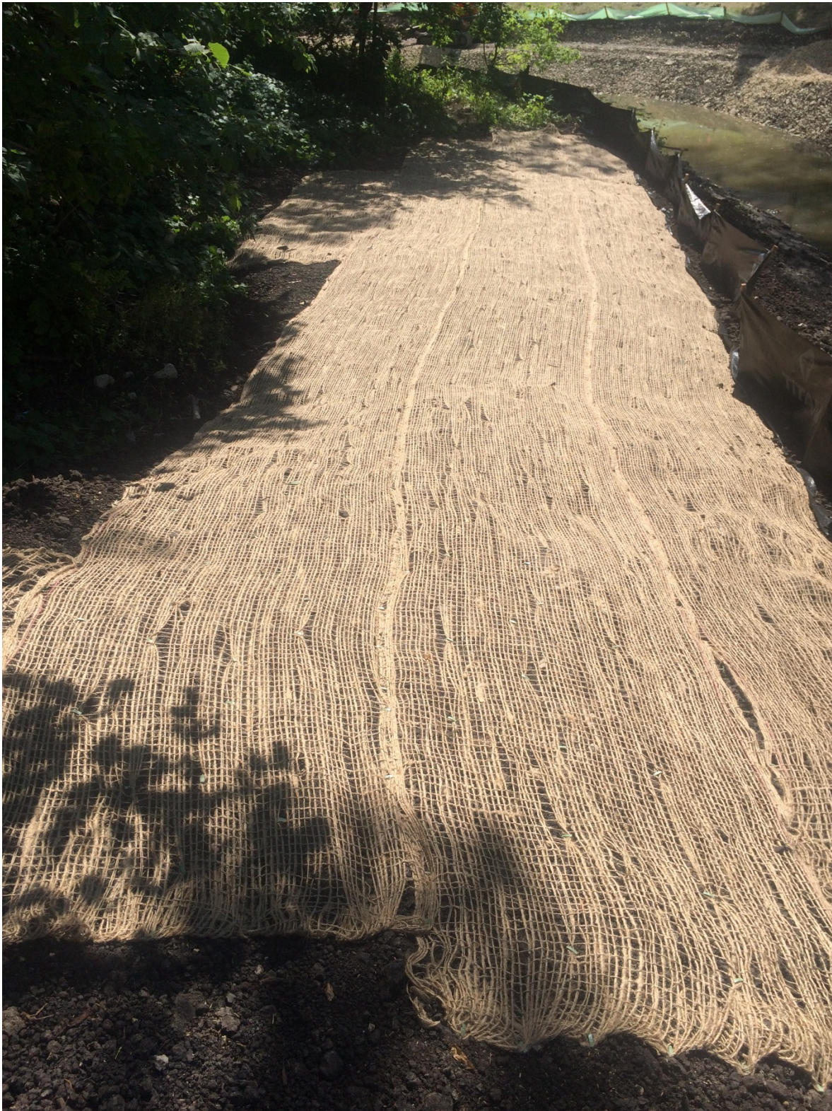
Photo 8 - Erosion control blanket placed on seeded topsoil at 3154 Henderson Highway.
