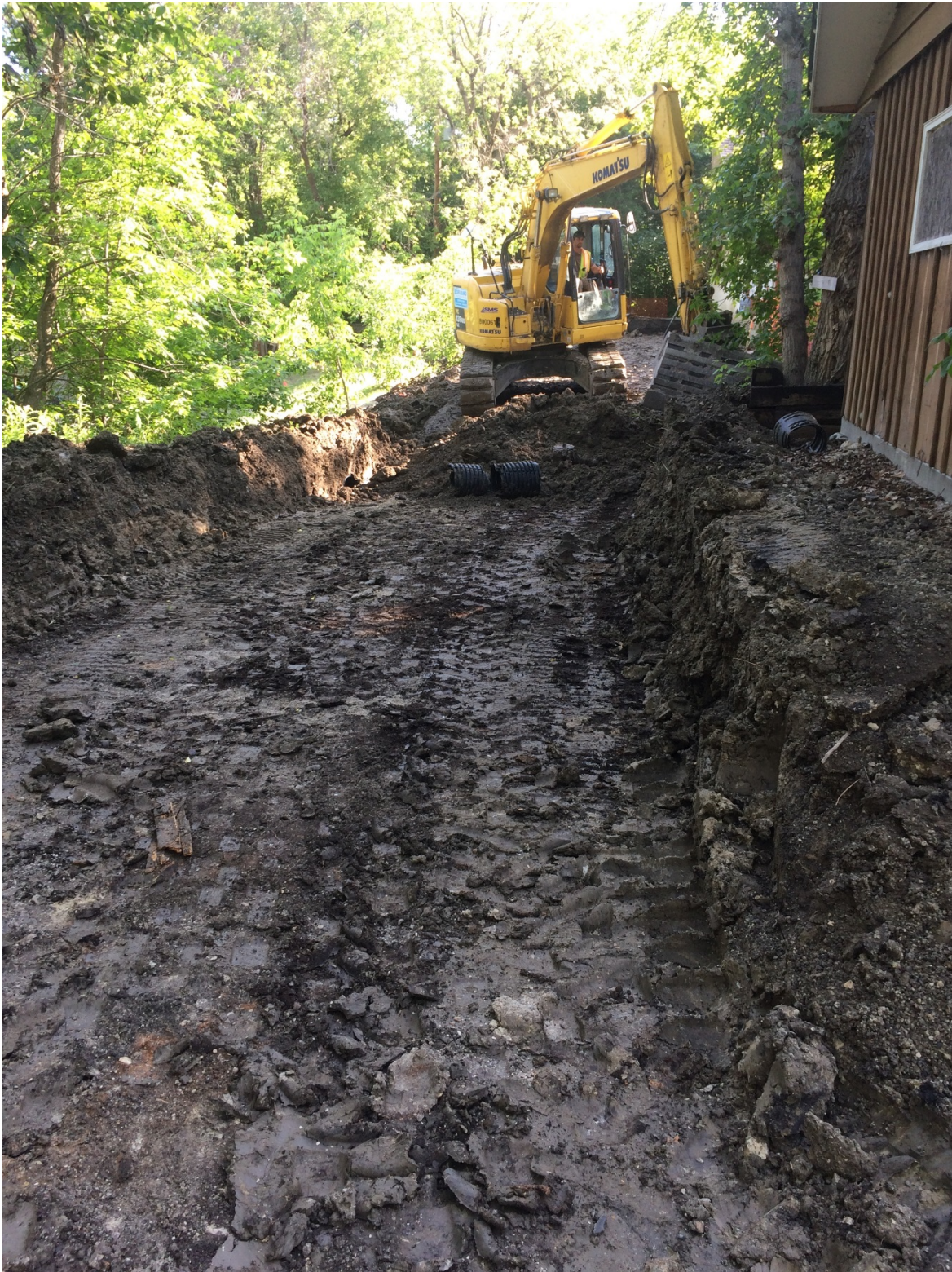
Photo 5 - Removal of organics below original dike at 3144 Henderson Highway.
