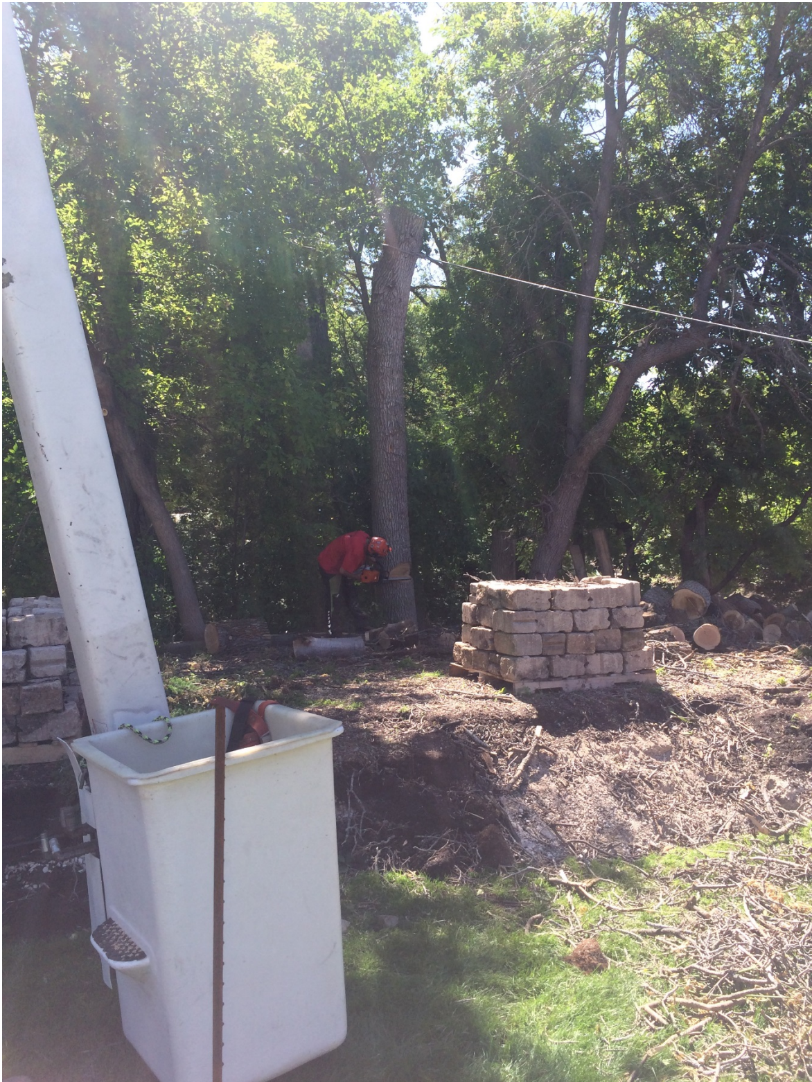
Photo 9 - Arborists removing select trees at 1020 Highland Park Drive.
