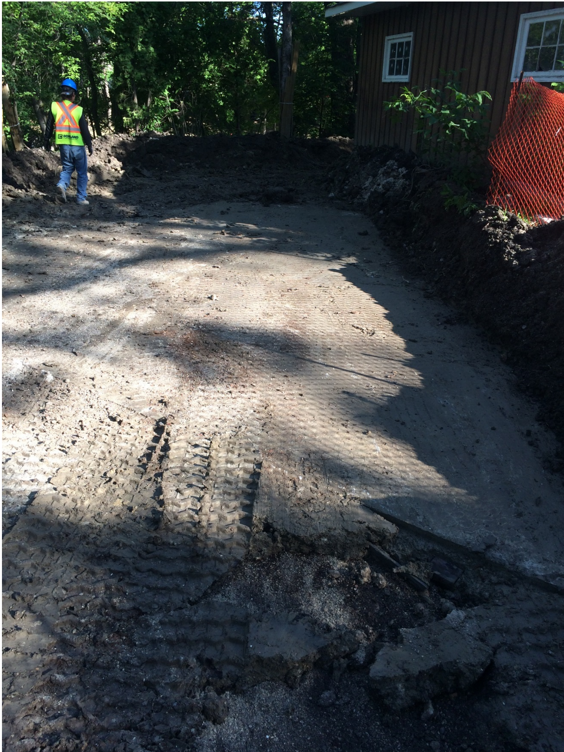
Photo 2 - Concrete garage pad below footprint of dike at 3144 Henderson Highway.
