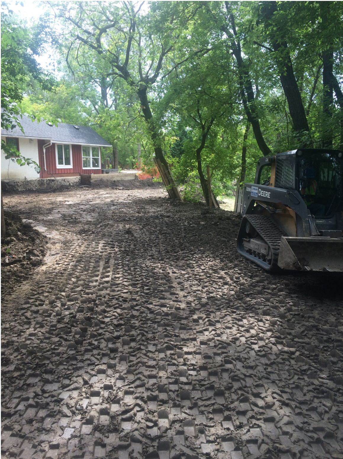
Photo 7 - Placement of new clay fill at 3144 Henderson Highway.
