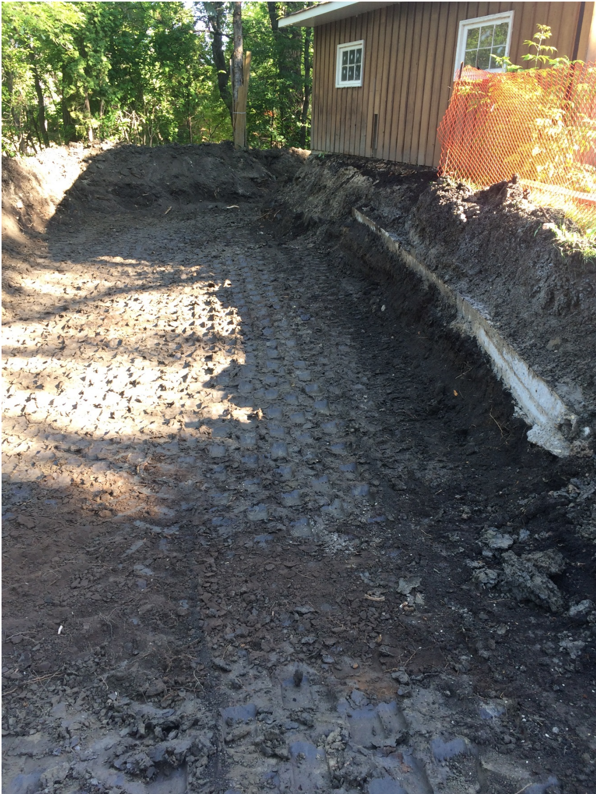
Photo 4 - Concrete garage pad removed at 3144 Henderson Highway.
