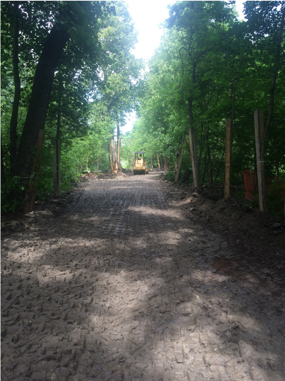
Photo 6 - Placement of new clay fill at 3154 Henderson Highway.
