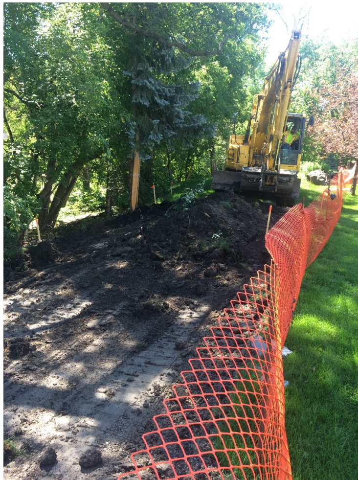
Photo 1 - Removal of the existing dike at 1030 Highland Park Drive.
