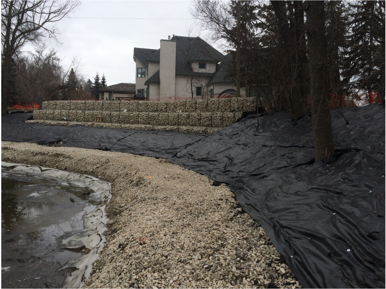
Photo 8 - Non-woven geotextile placed on topsoil at 1030 Highland Park Drive.
