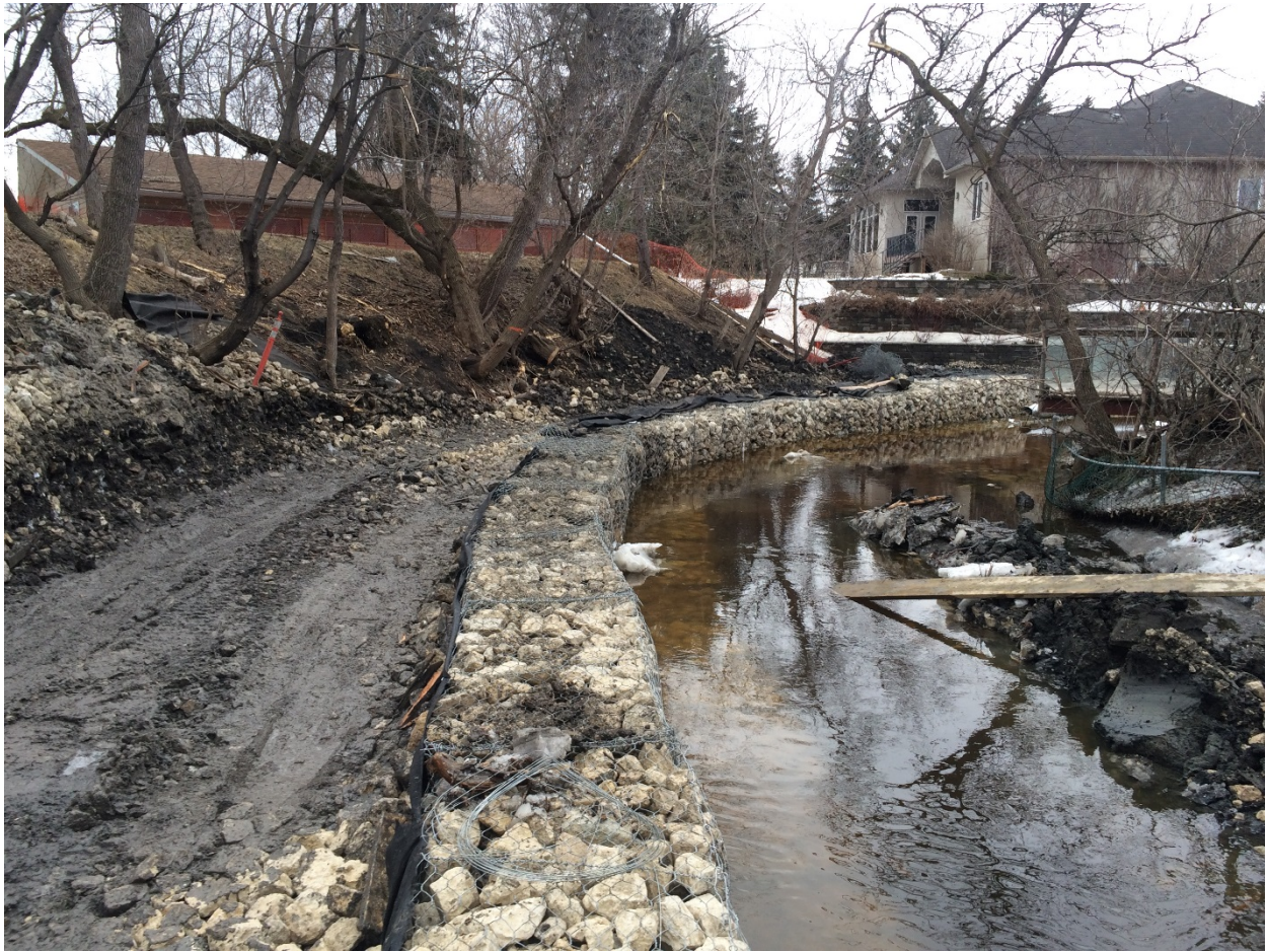
Photo 12 - Completed gabion baskets at 3144 Henderson Highway.
