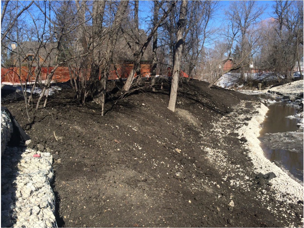
Photo 3 - Topsoil and terrace rock placed at 1040 Highland Park Drive.
