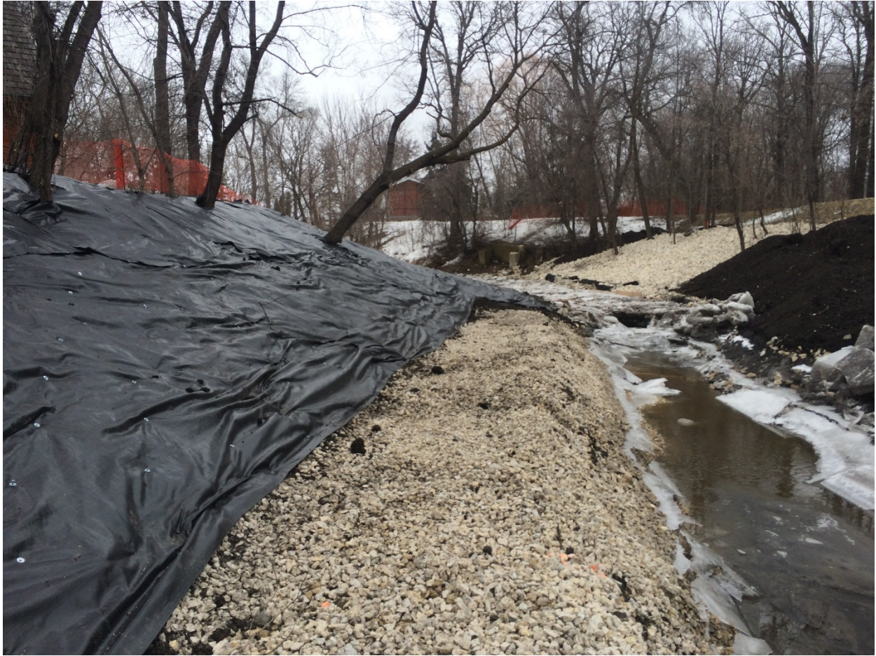
Photo 7 - Non-woven geotextile placed on topsoil at 1040 Highland Park Drive.
