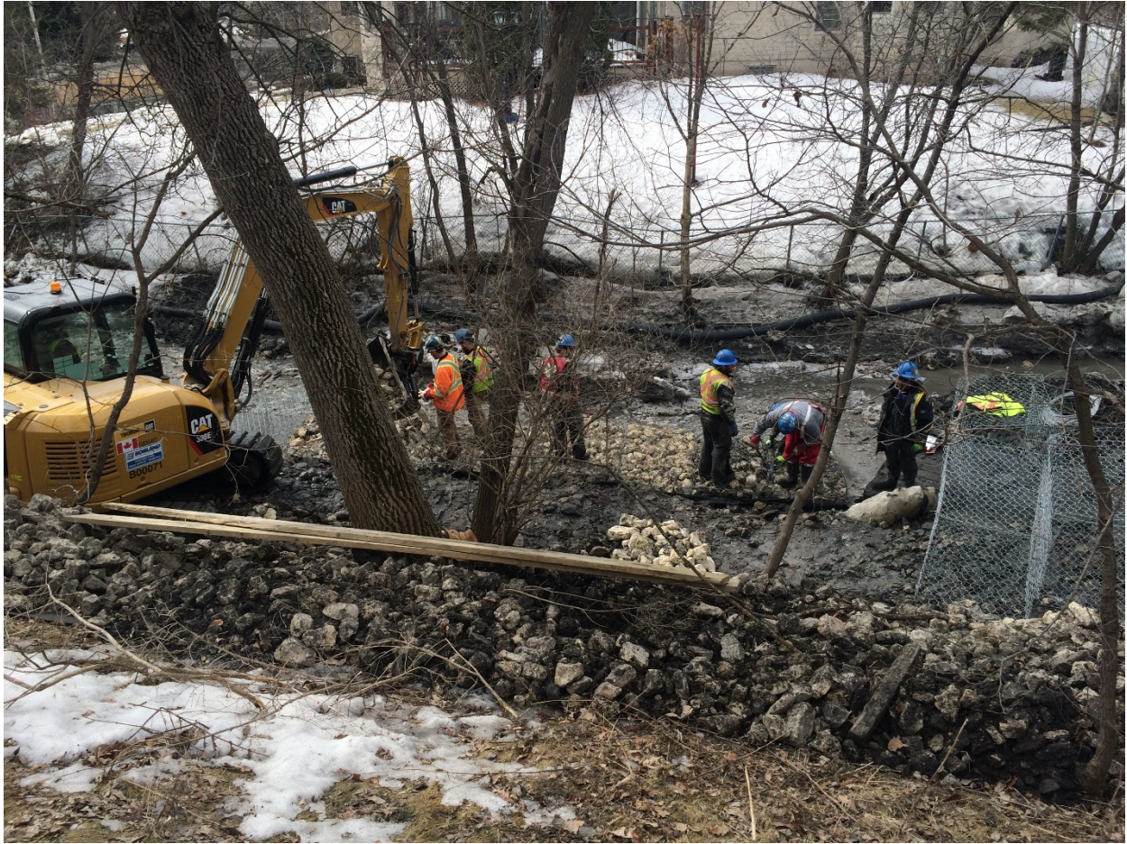
Photo 11 - Gabion basket filling at 3144 Henderson Highway.
