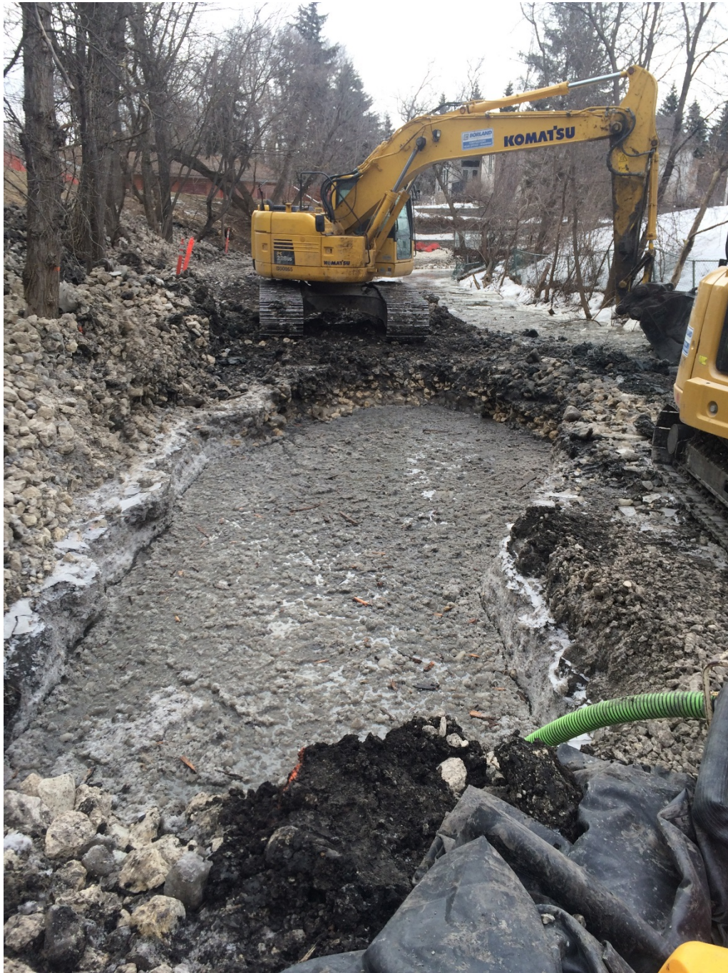
Photo 10 - Shear key excavation at 3144 Henderson Highway.
