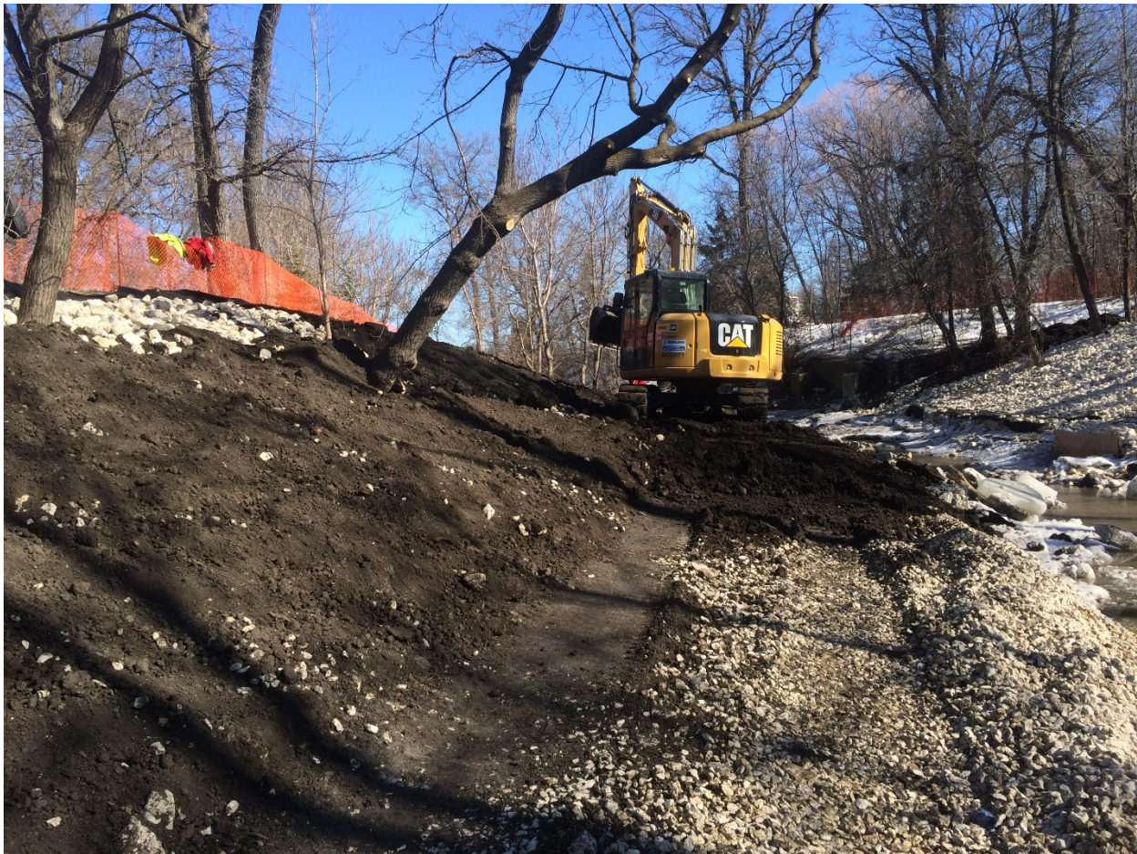
Photo 1 - Topsoil placement at 1040 Highland Park Drive.
