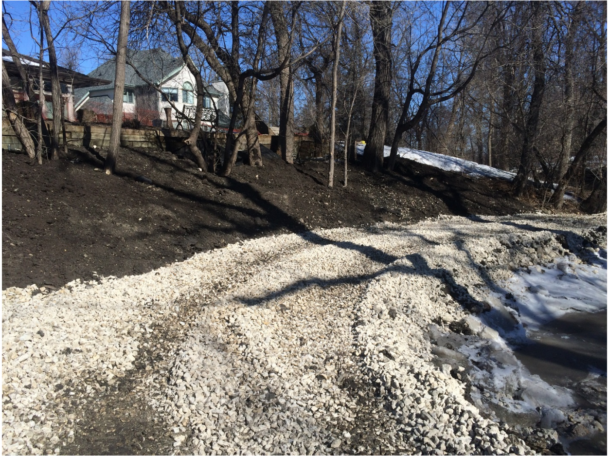
Photo 5 - Topsoil and terrace rock placed at 1020 Highland Park Drive.
