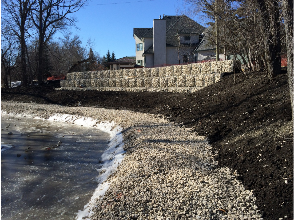
Photo 4 - Topsoil and terrace rock placed at 1030 Highland Park Drive.
