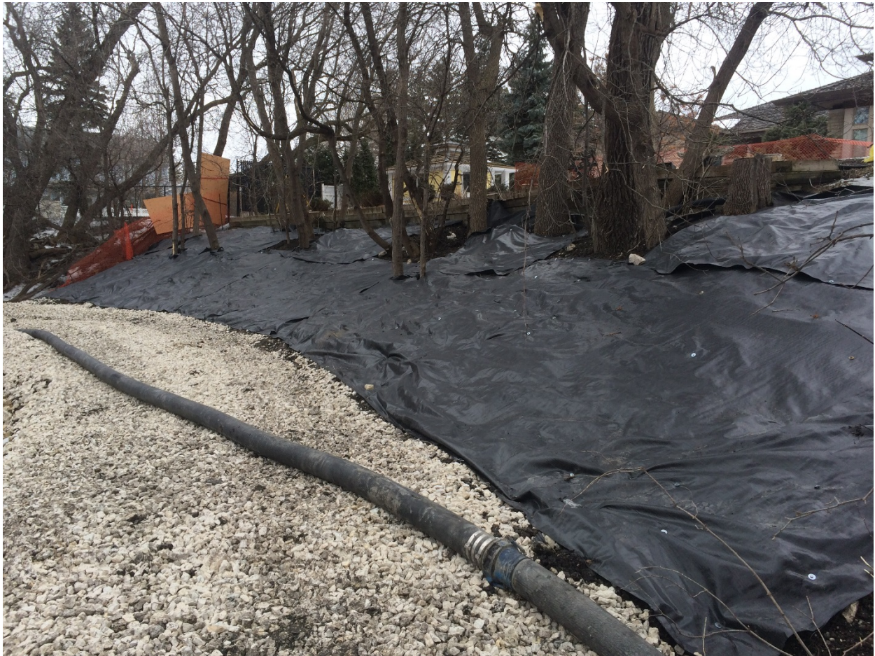
Photo 9 - Non-woven geotextile placed on topsoil at 1020 Highland Park Drive.
