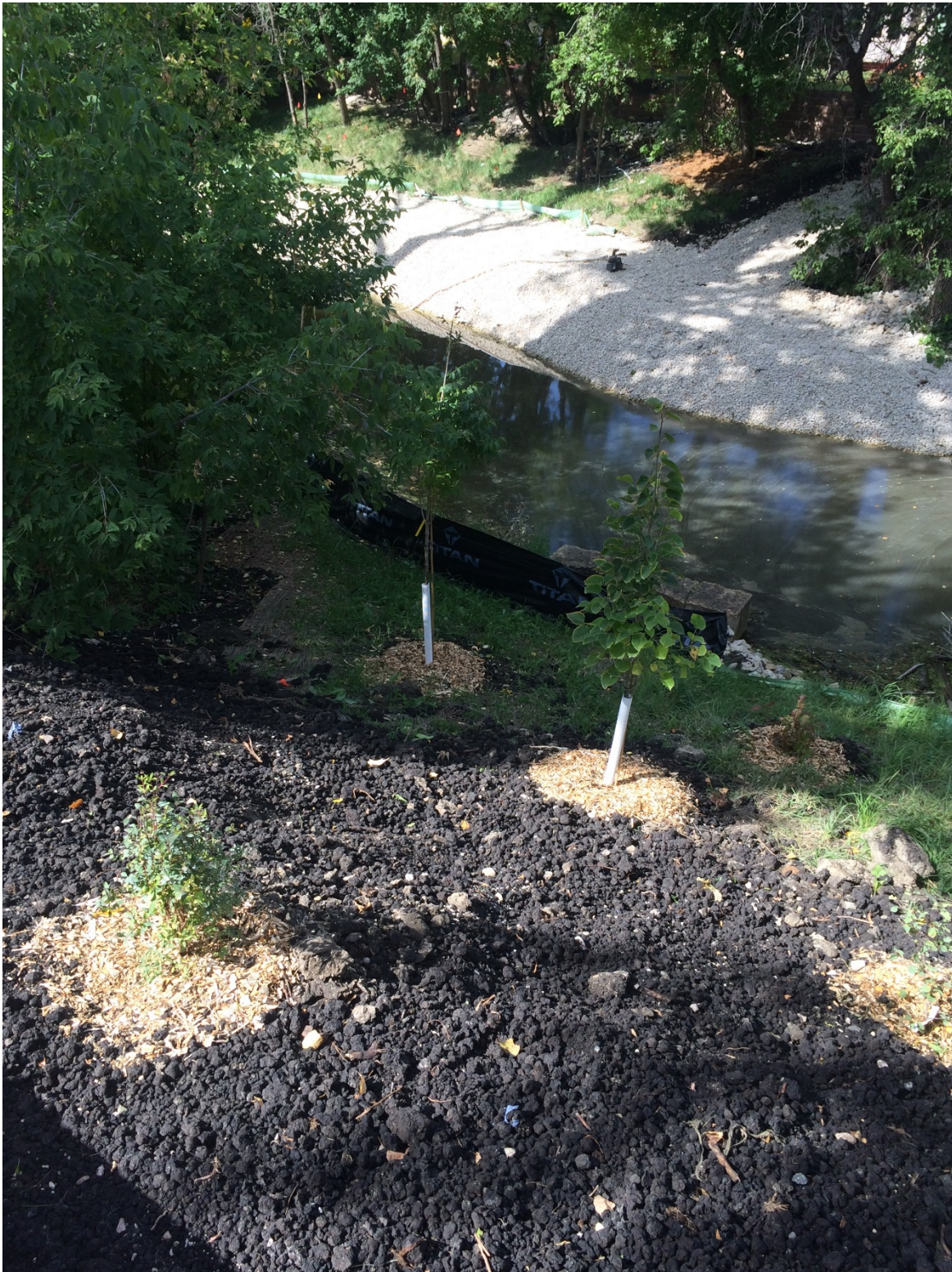
Photo 5 - New trees and shrubs planted on rockfill toe berm.
