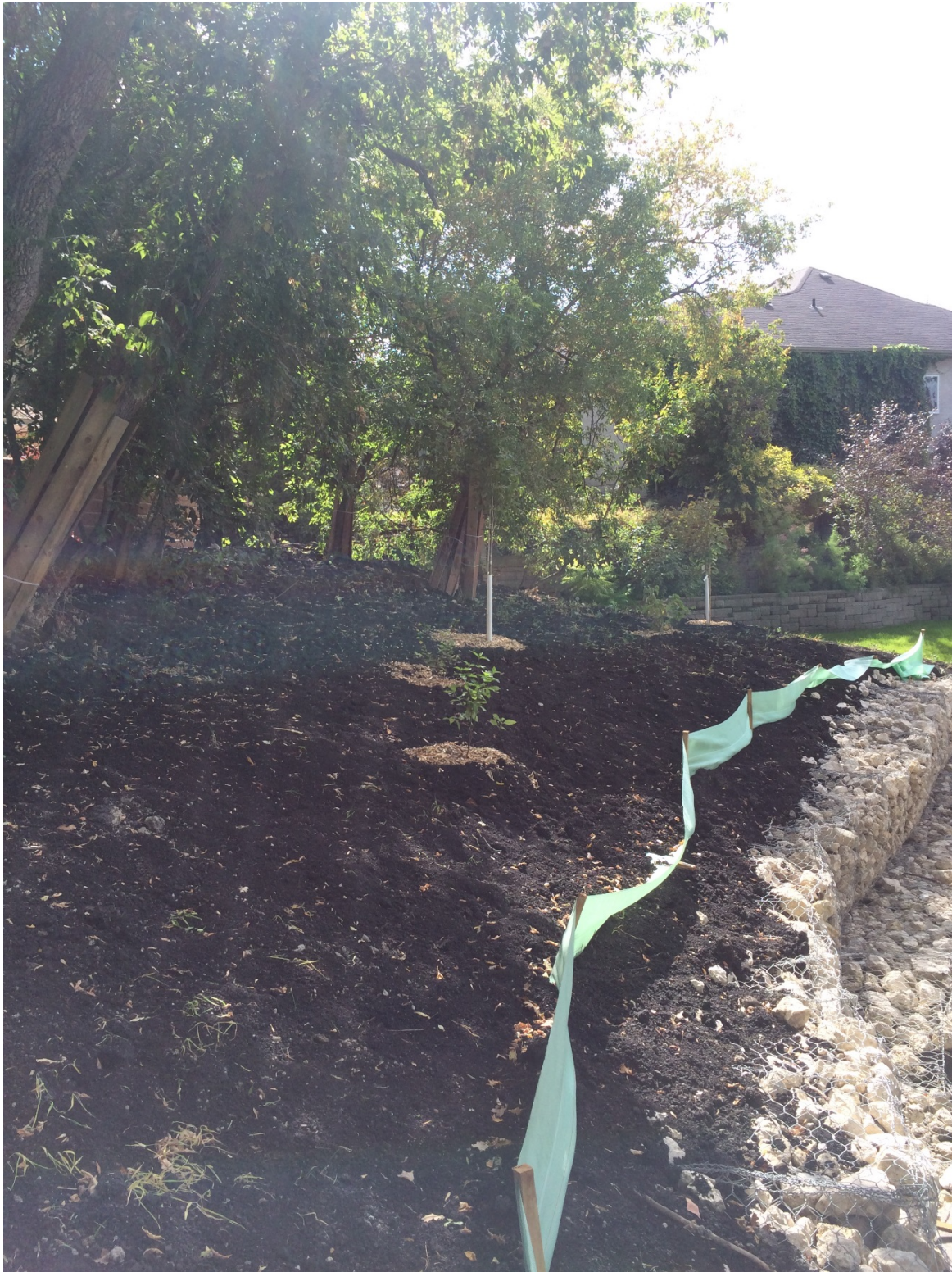
Photo 3 - New trees and shrubs planted on rockfill toe berm.
