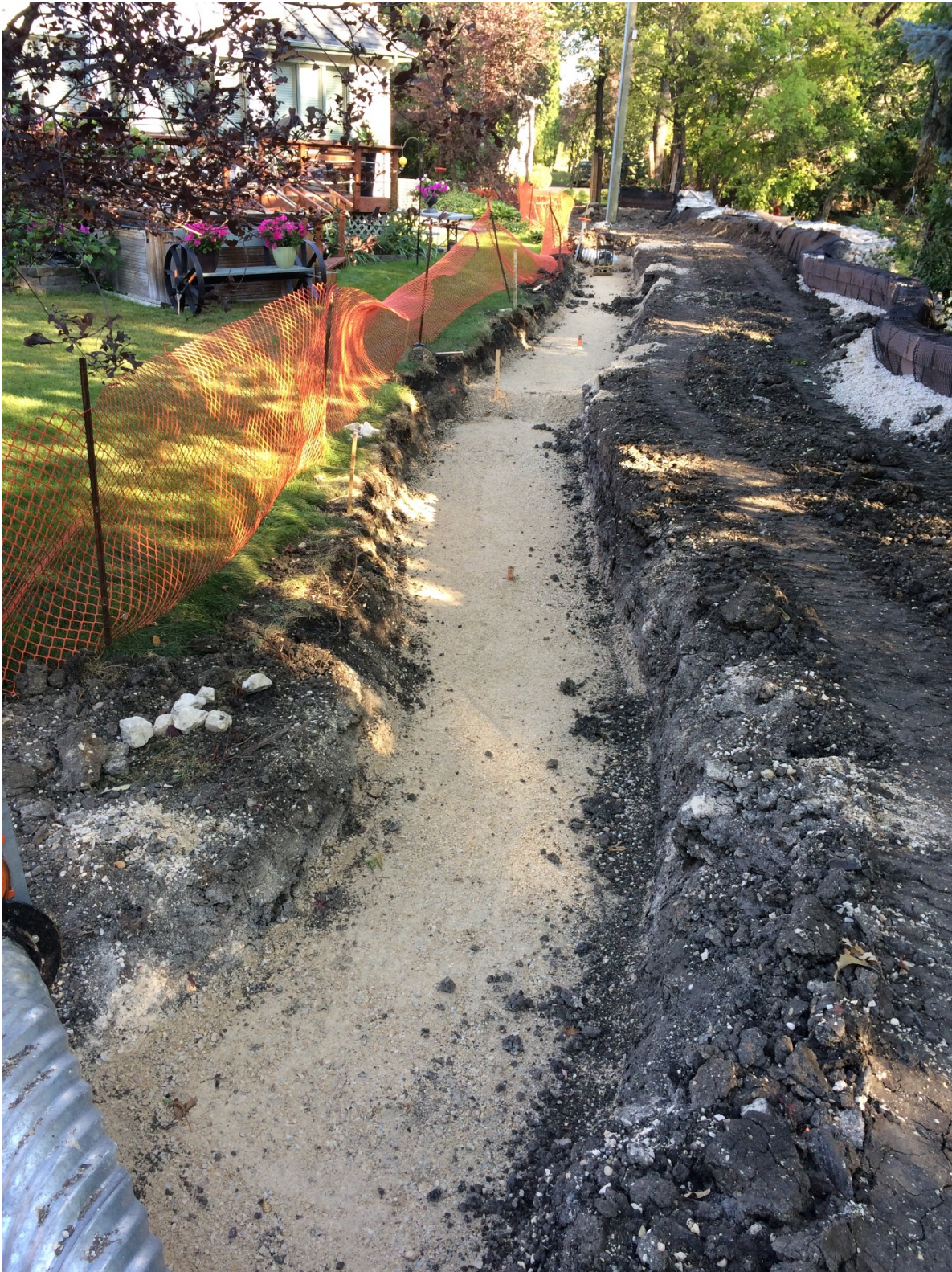
Photo 2 - Foundation for house side segmental block wall at 1030 Highland Park Drive.
