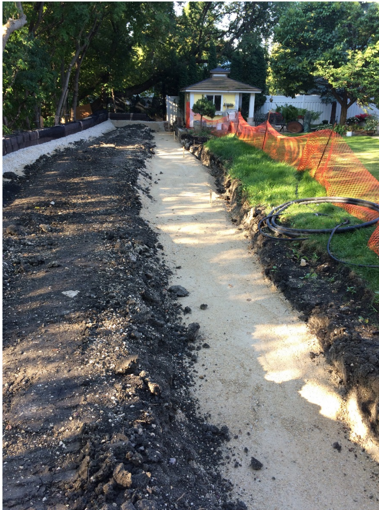
Photo 1 - Foundation for house side segmental block wall at 1020 Highland Park Drive.
