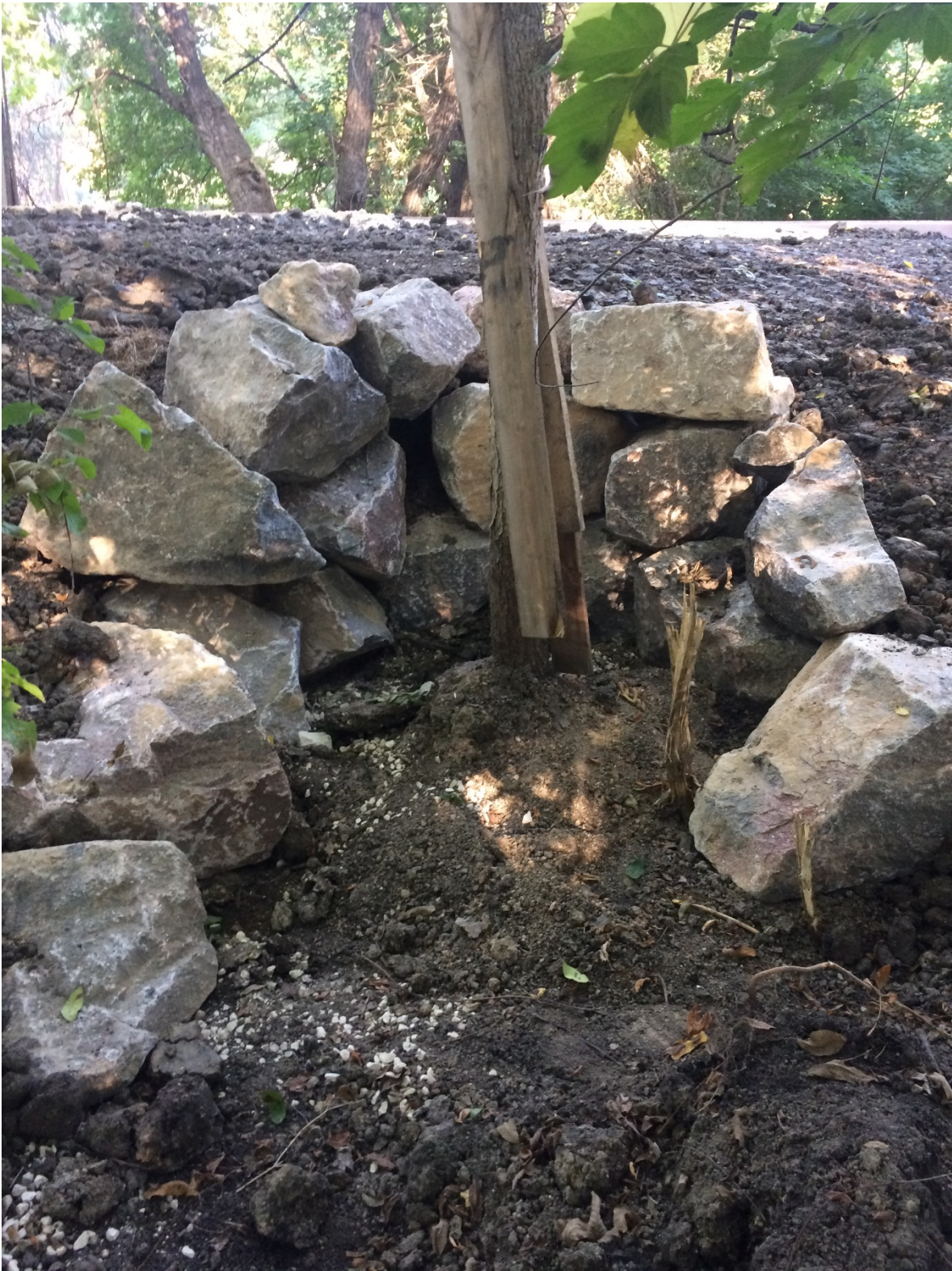
Photo 7 - Tree well at 3154 Henderson Highway.
