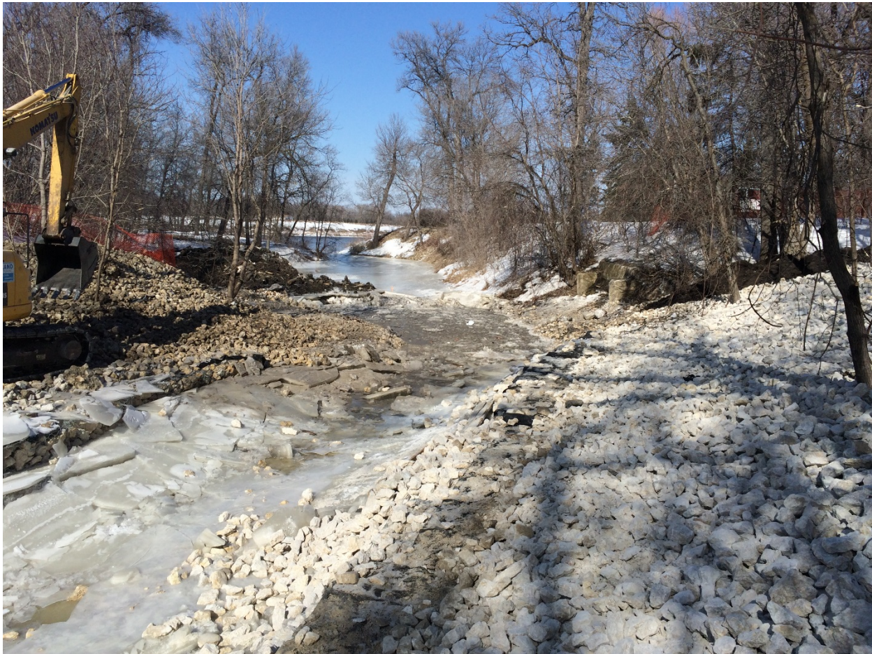
Photo 4 - Cofferdam removed between 1040 Highland Park Drive and 3154 Henderson Highway.
