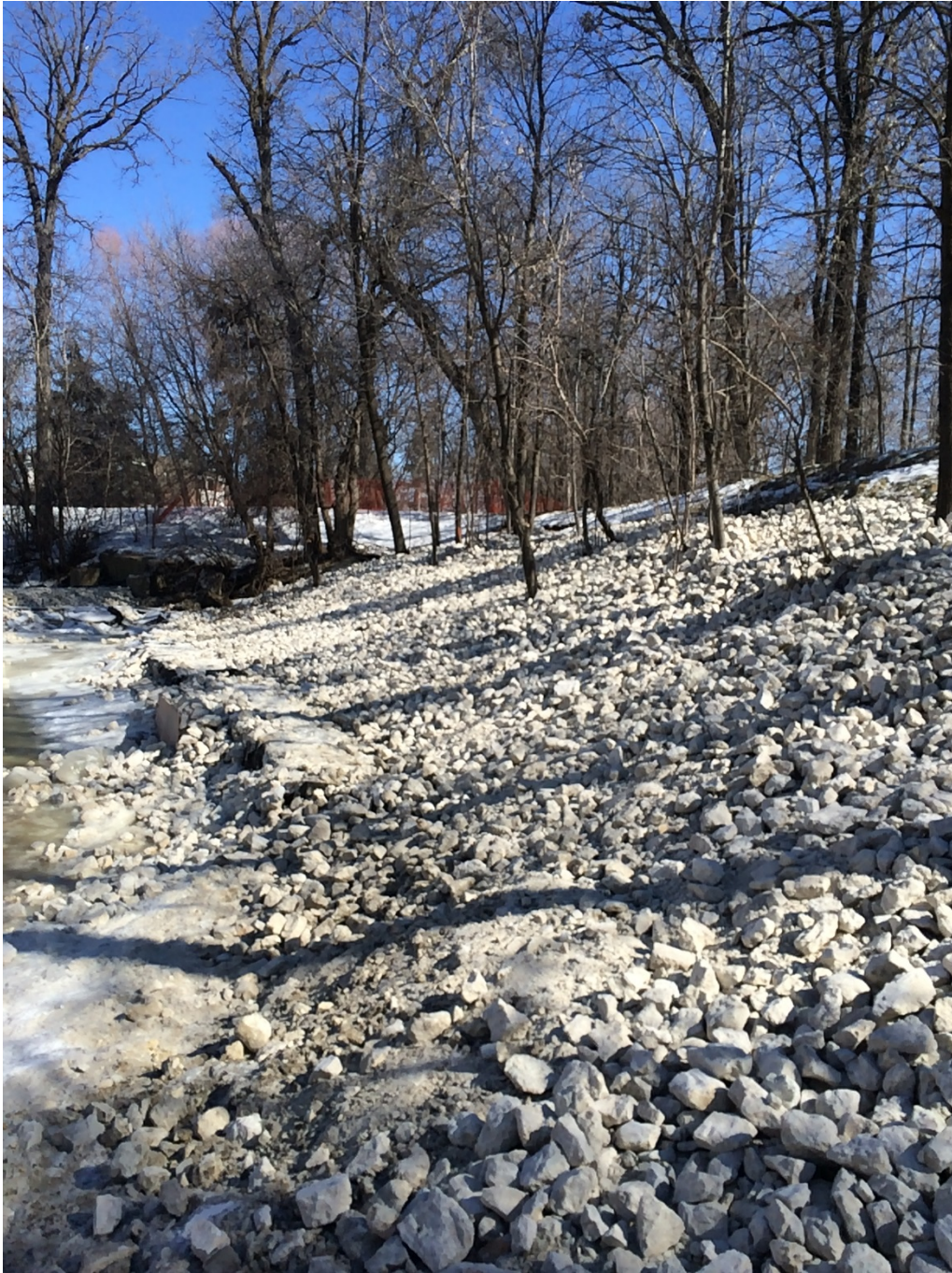
Photo 3 - Shaped rockfill toe berm at 3154 Henderson Highway.
