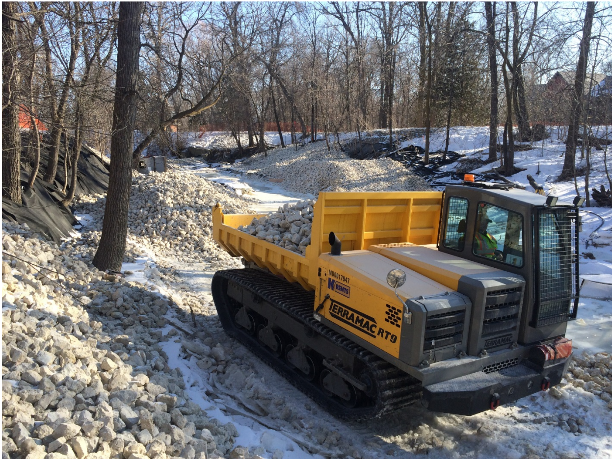
Photo 1 - Hauling rockfill for toe berm at 1040 Highland Park Drive.
