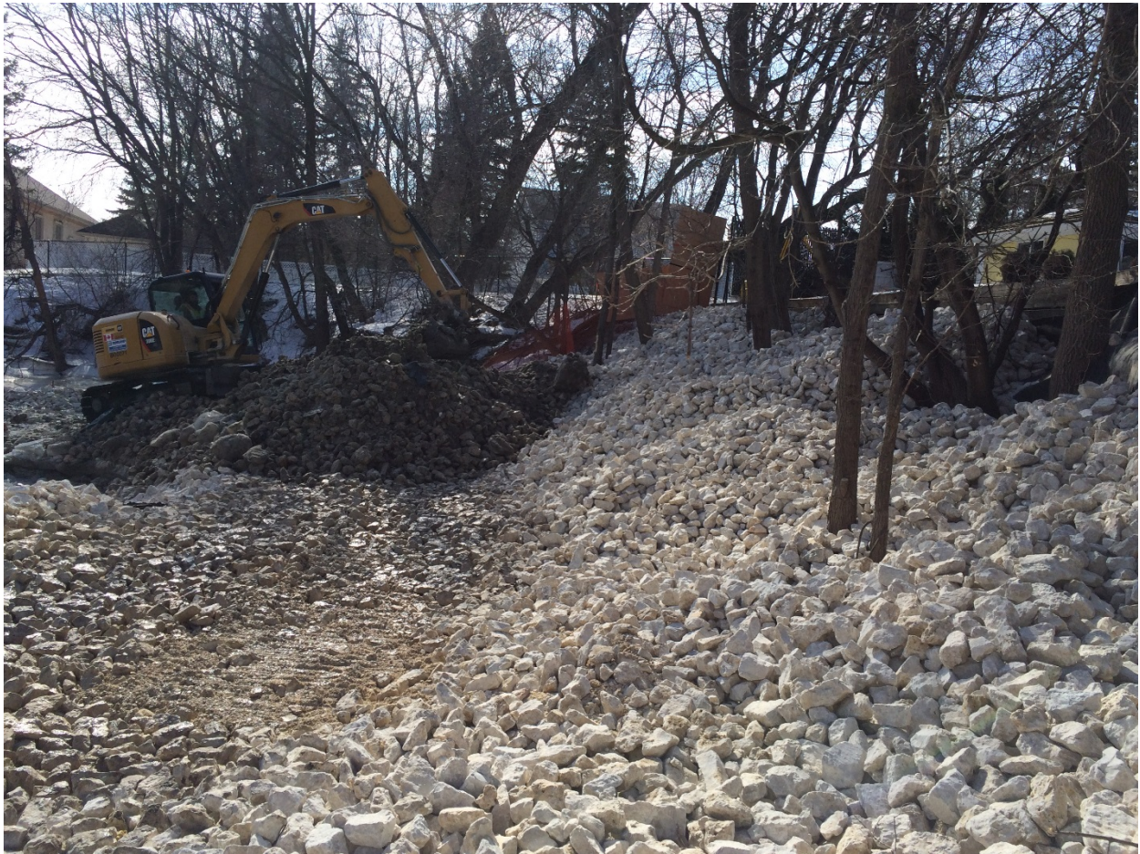
Photo 5 - Rockfill toe berm placement at 1020 Highland Park Drive.
