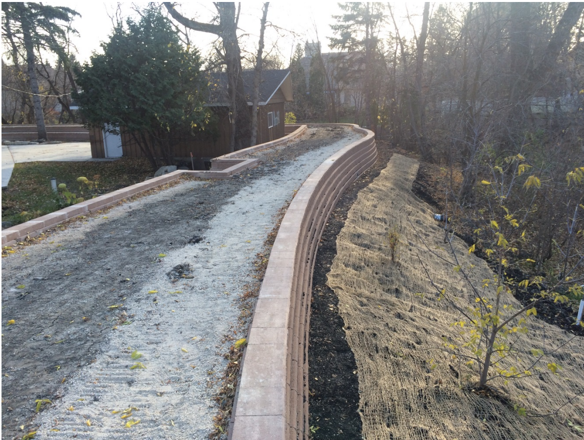
Photo 1 - Dike at 3144 Henderson Highway.
