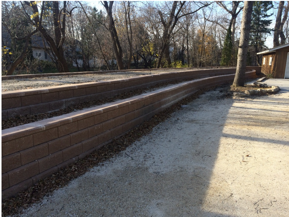
Photo 6 - Dike at 3144 Henderson Highway.
