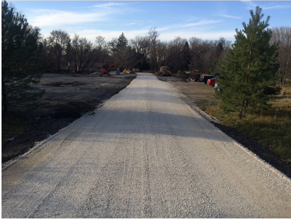
Photo 4 - Access roadway at 3144 Henderson Highway.
