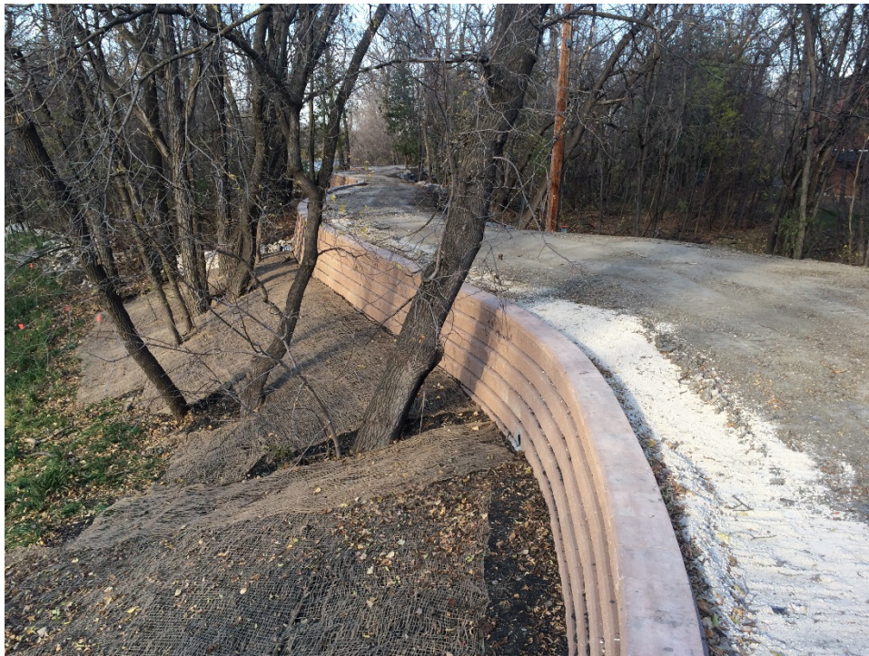
Photo 3 - Dike at 3144/3154 Henderson Highway.
