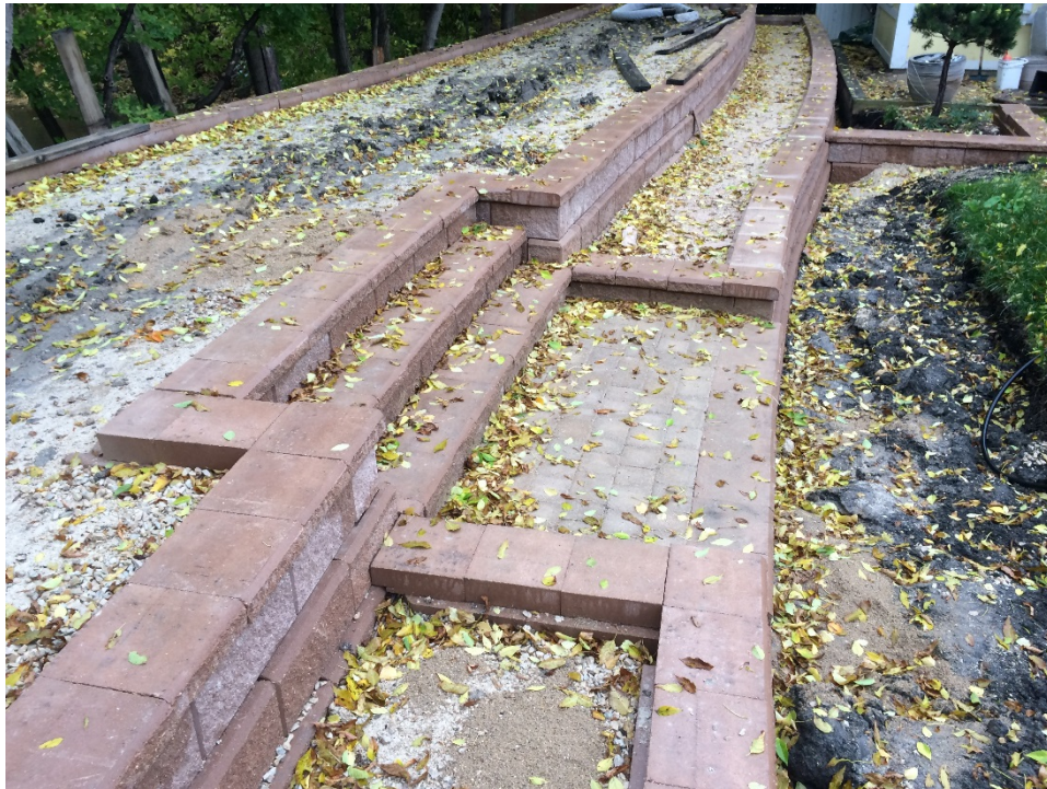
Photo 8 - Stairs at 1020 Highland Park Drive.
