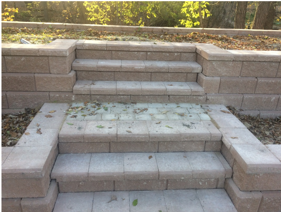
Photo 7 - Stairs at 1040 Highland Park Drive.
