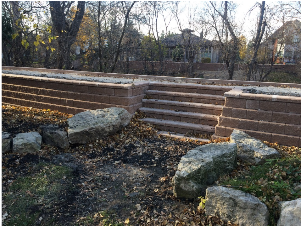
Photo 2 - Stairs at 3144 Henderson Highway.
