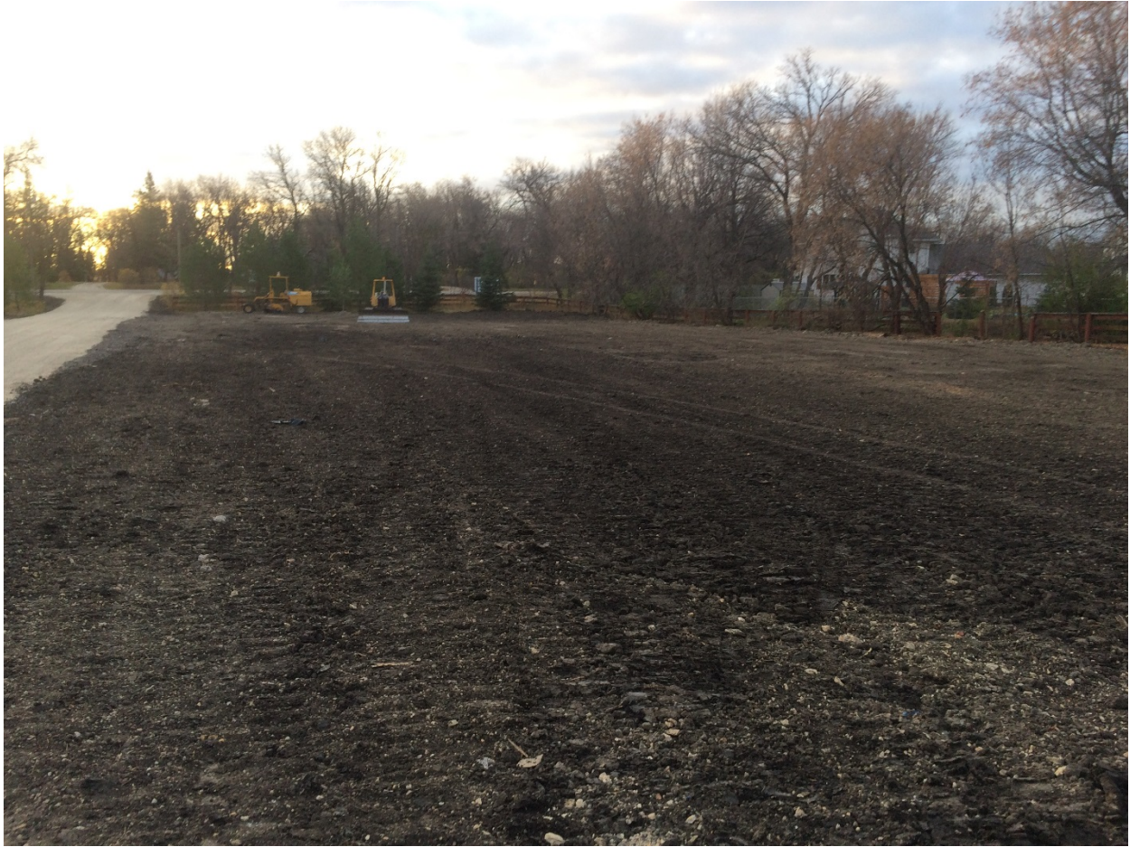
Photo 10 - Site laydown area at 3144 Henderson Highway.
