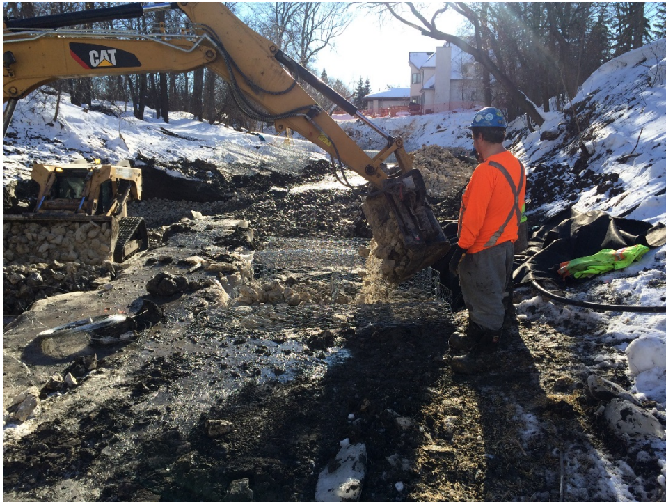
Photo 2 - Gabion basket filling at 1040 Highland Park Drive.
