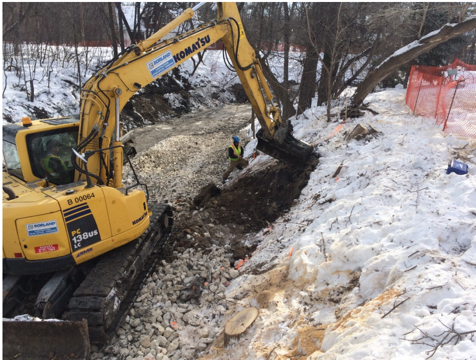
Photo 5 - Excavation for gabion basket placement at 1030 Highland Park Drive.
