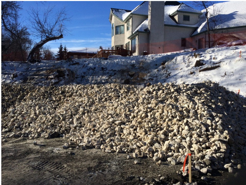
Photo 3 - Rockfill toe berm placement at 1030 Highland Park Drive.
