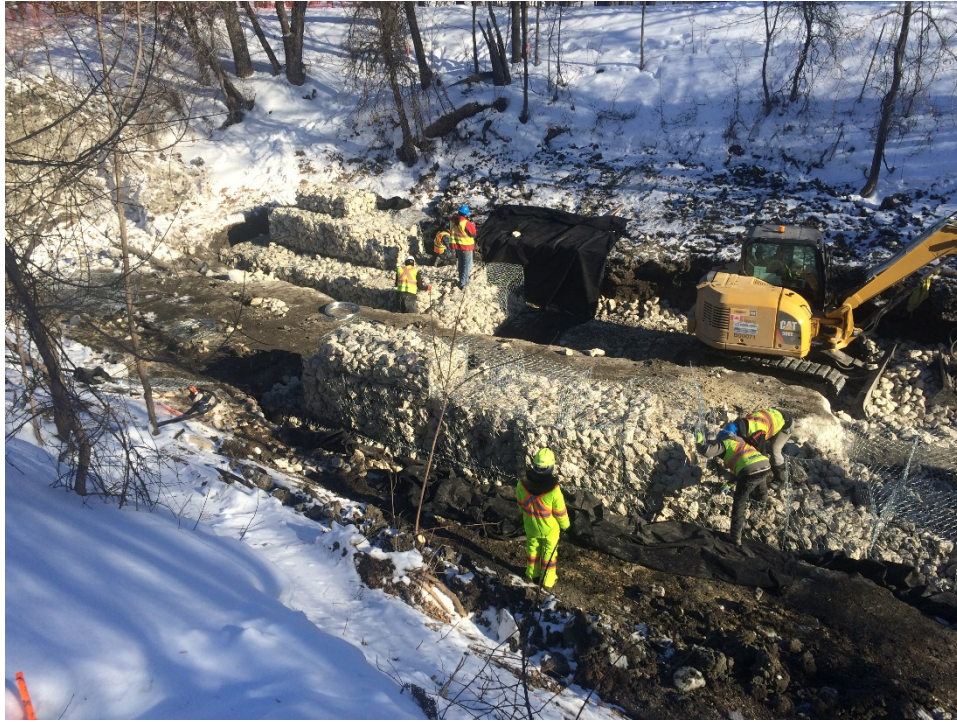
Photo 4 - Gabion basket installation at 1040 Highland Park Drive and 3154 Henderson Highway.
