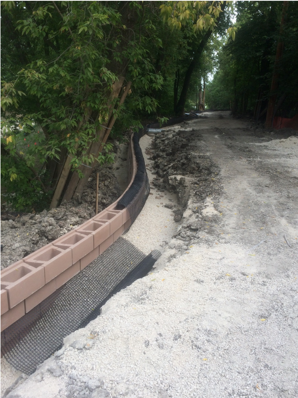
Photo 13 - Placement of the segmental block wall at 3144 and 3154 Henderson Highway.
