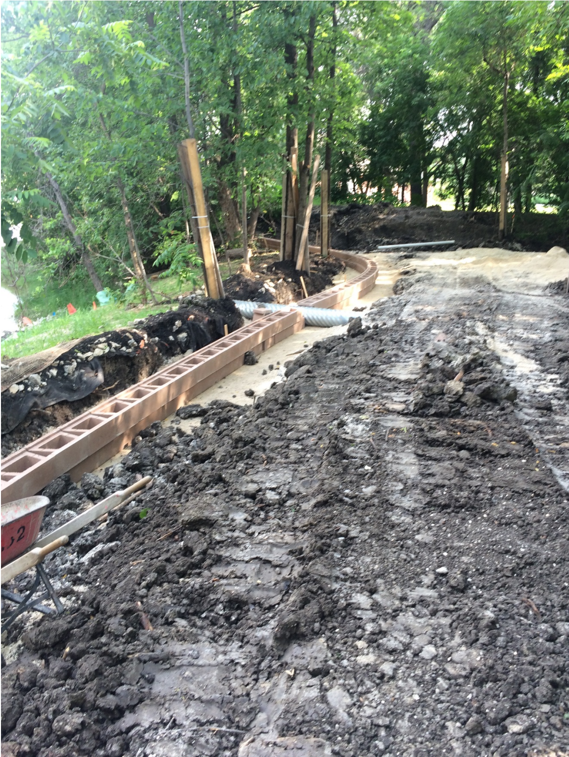
Photo 7 - Placement of the segmental block wall at 3154 Henderson Highway.
