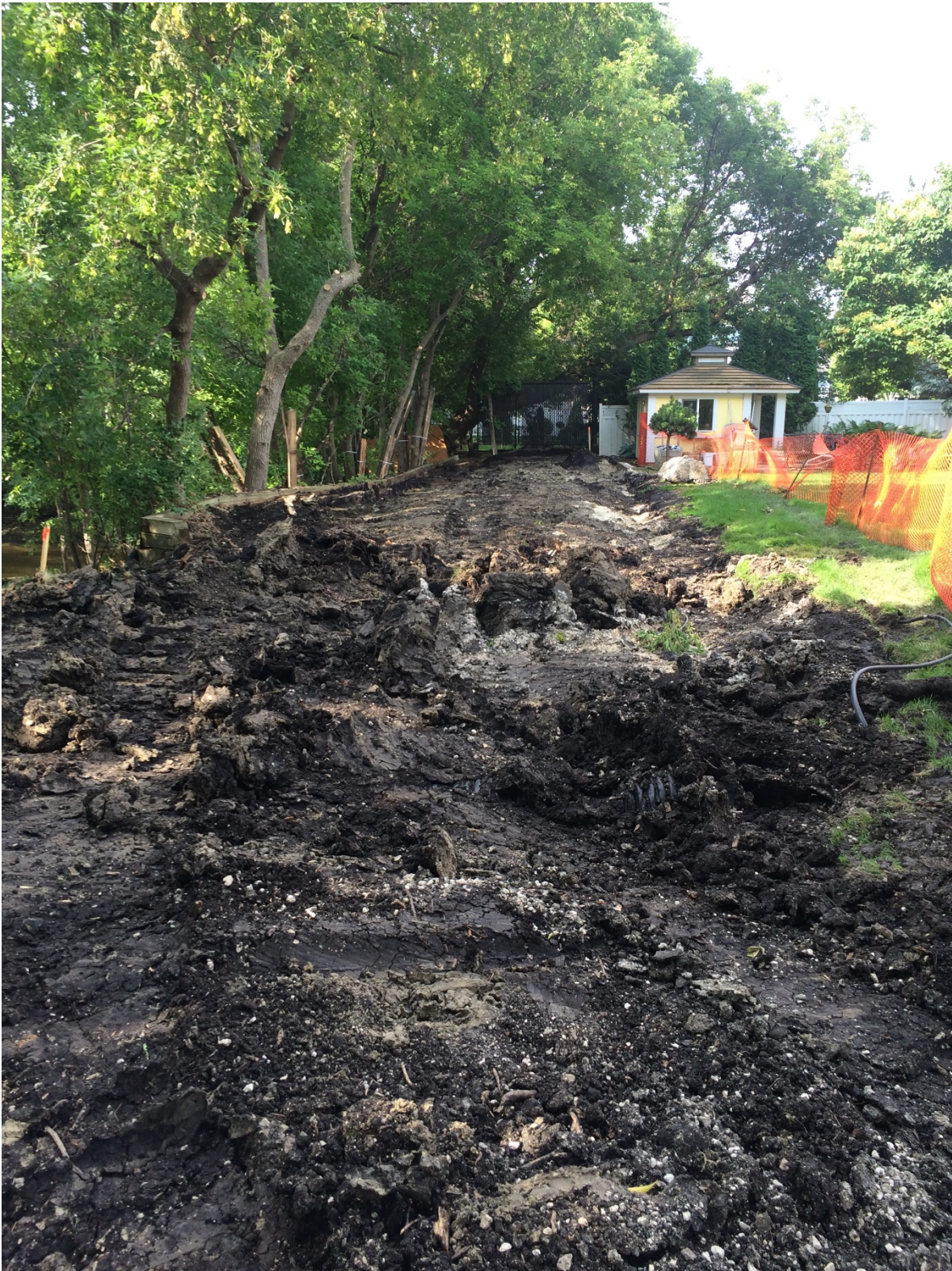
Photo 3 - Removal of existing dike at 1020 Highland Park Drive.
