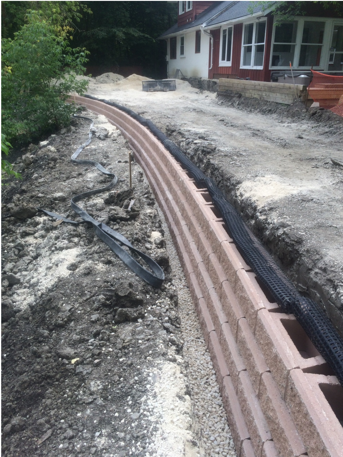
Photo 14 - Placement of the segmental block wall at 3144 Henderson Highway.
