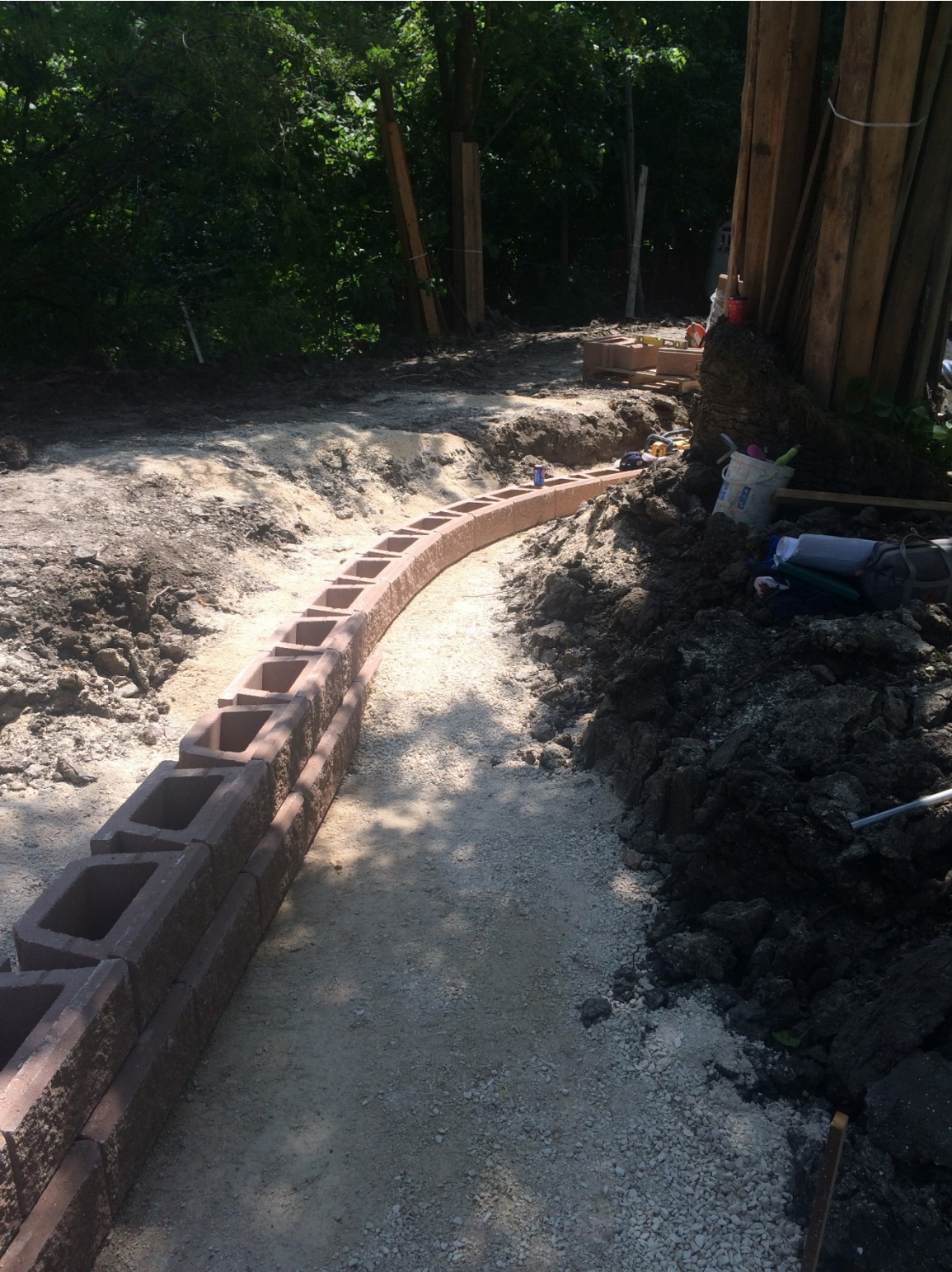
Photo 8 - Placement of the segmental block wall at 3154 Henderson Highway.
