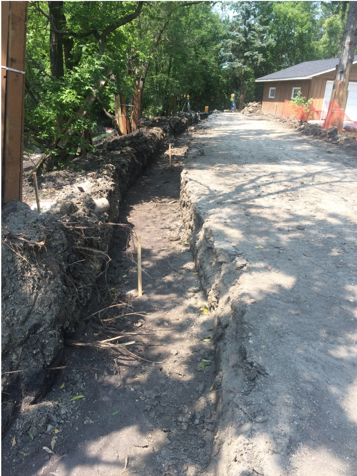
Photo 4 - Foundation for creek side segmental block wall excavated at 3144 Henderson Highway.
