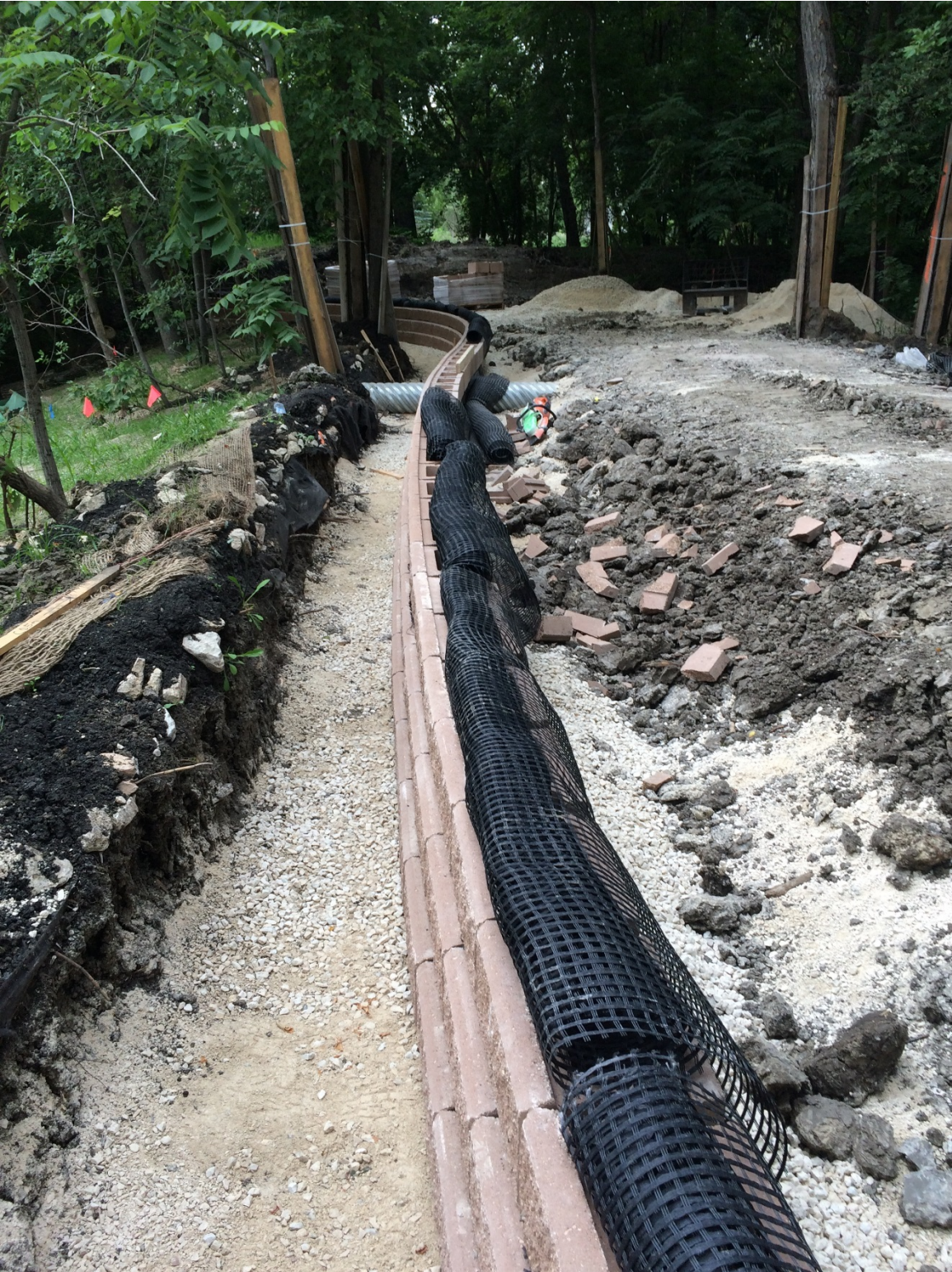
Photo 11 - Placement of the segmental block wall at 3154 Henderson Highway.
