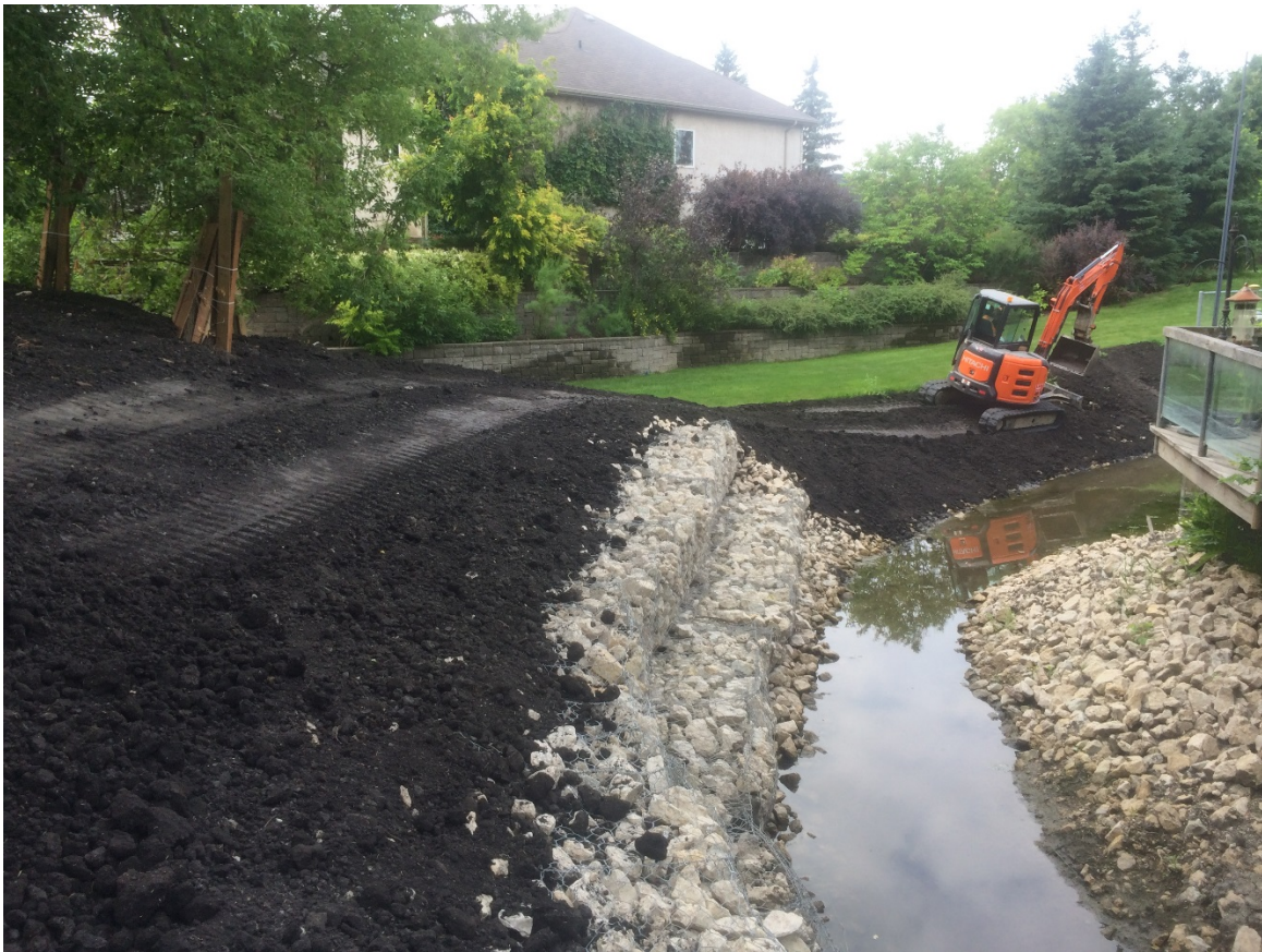
Photo 1 - Topsoil placement on the rockfill toe berm at 3144 Henderson Highway.
