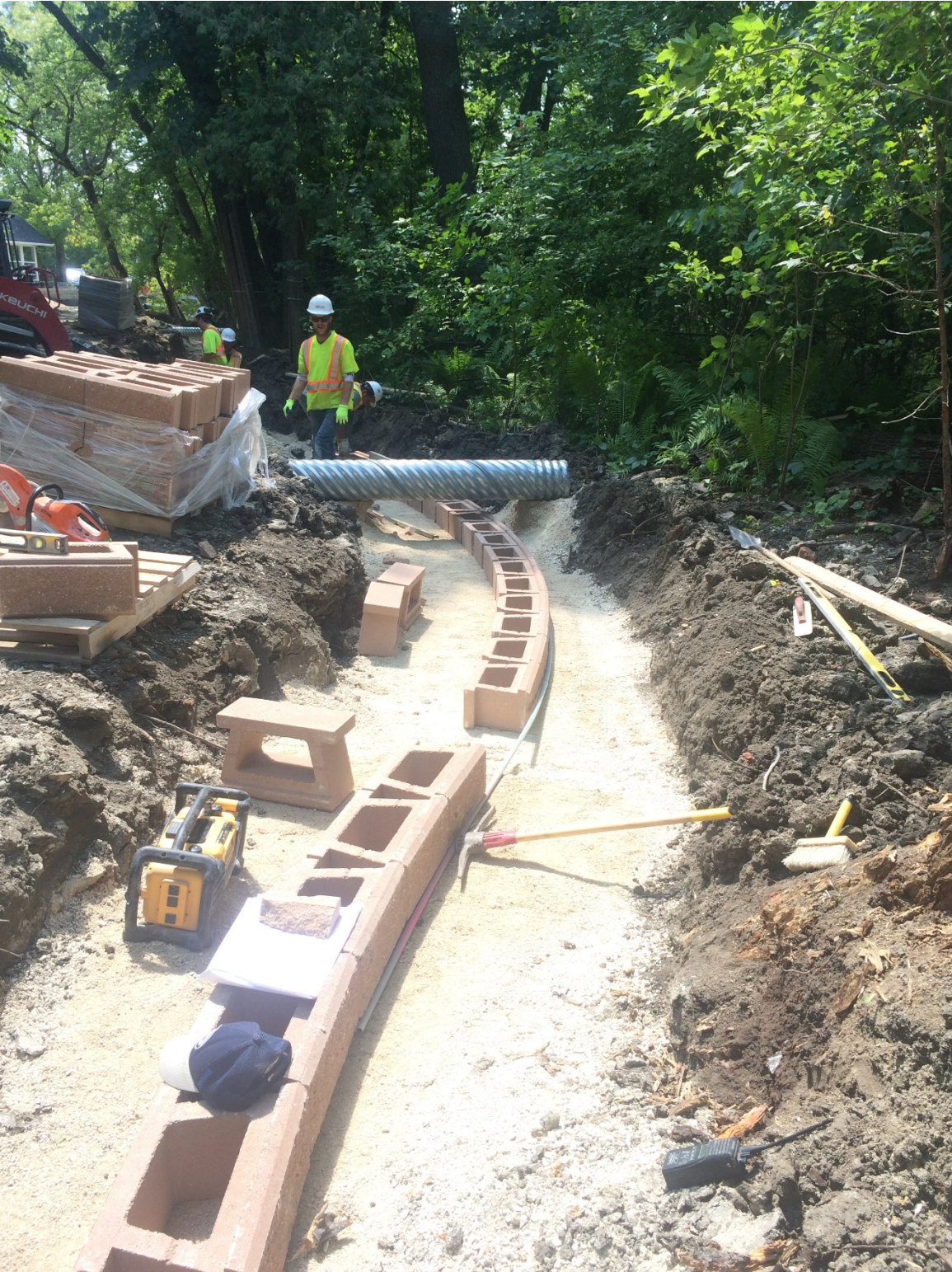
Photo 9 - Placement of the segmental block wall at 3154 Henderson Highway.
