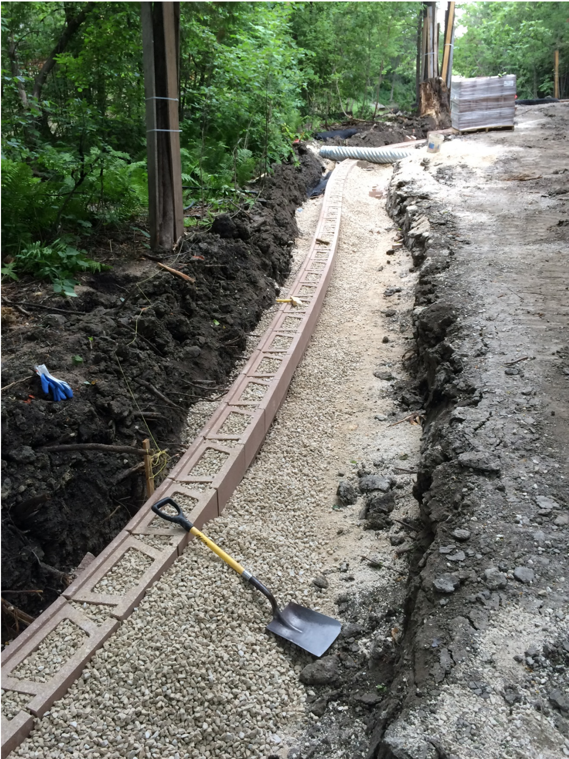
Photo 12 - Placement of the segmental block wall at 3154 Henderson Highway.
