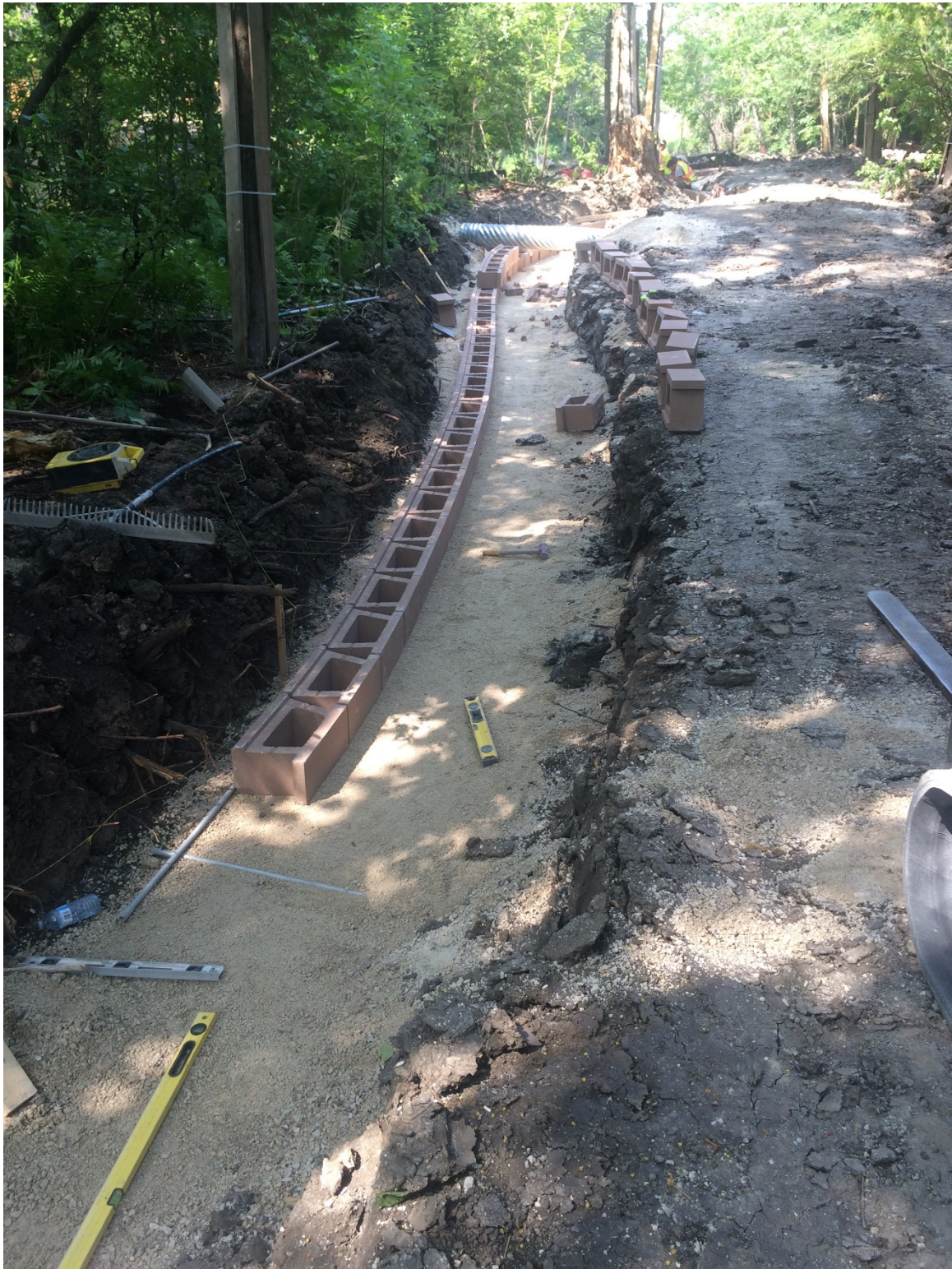
Photo 10 - Placement of the segmental block wall at 3154 Henderson Highway.
