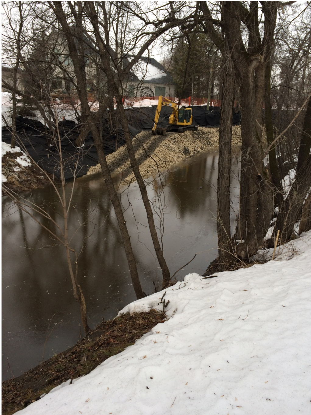
Photo 2 - Increased water level at 1030 Highland Park Drive.
