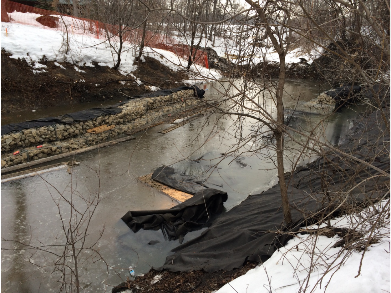
Photo 4 - Increased water level at 1040 Highland Park Drive and 3154 Henderson Highway.
