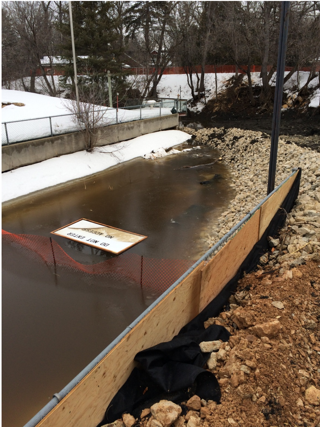
Photo 3 - Increased water level at Tartan Way culvert.
