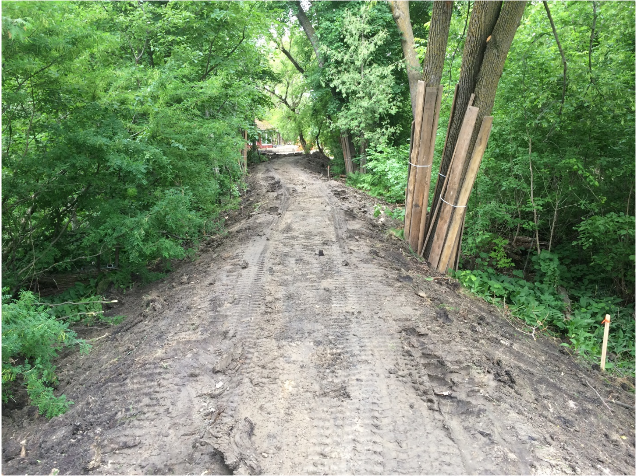
Photo 4 - Existing dike following the removal of organics at 3154 Henderson Highway, along with protected trees.
