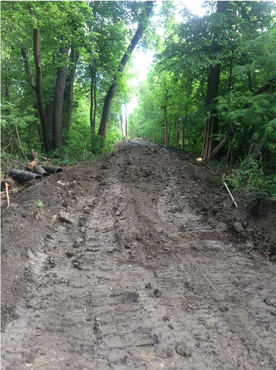
Photo 6 - Existing dike removal at 3154 Henderson Highway.
