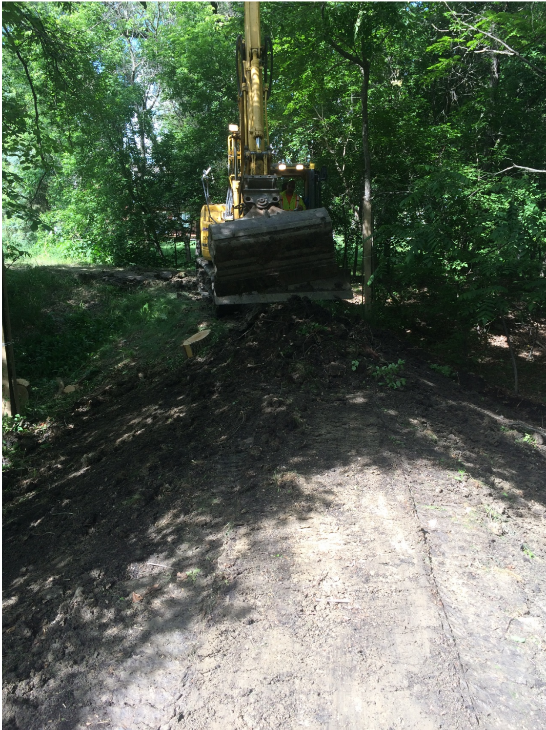
Photo 3 - Removal of organics from existing dike at 3154 Henderson Highway.
