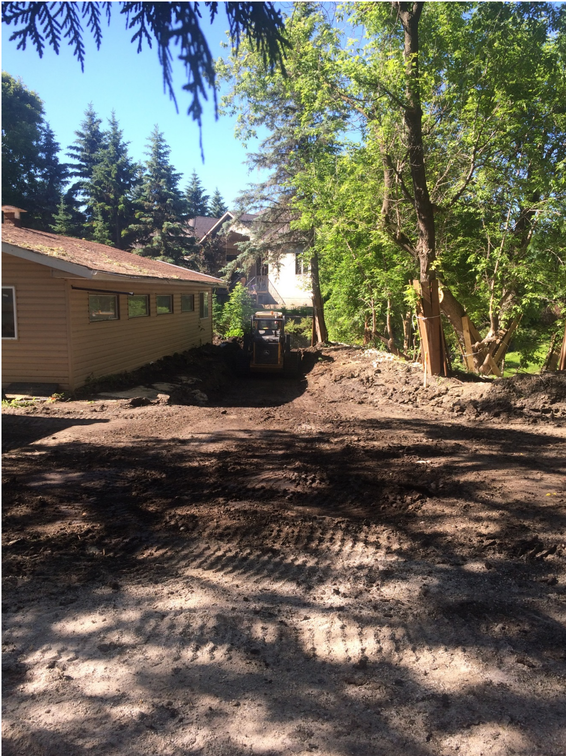
Photo 7 - Removal of organic material below existing dike at 3144 Henderson Highway.
