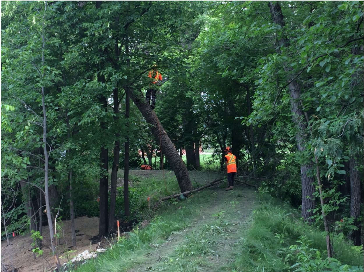
Photo 2 - Arborists pruning and removing trees at 3154 Henderson Highway.
