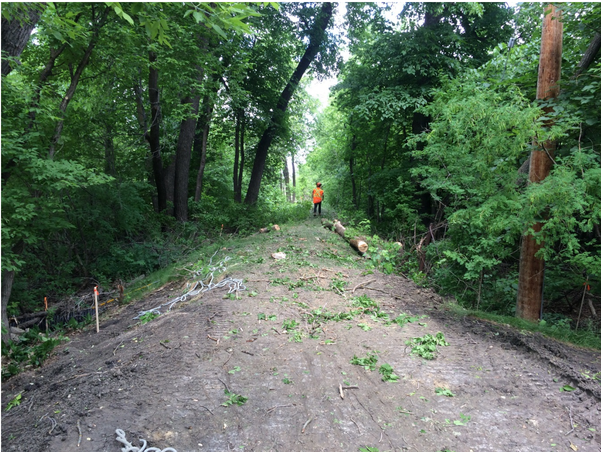
Photo 1 - Arborists pruning and removing trees at 3144 & 3154 Henderson Highway.
