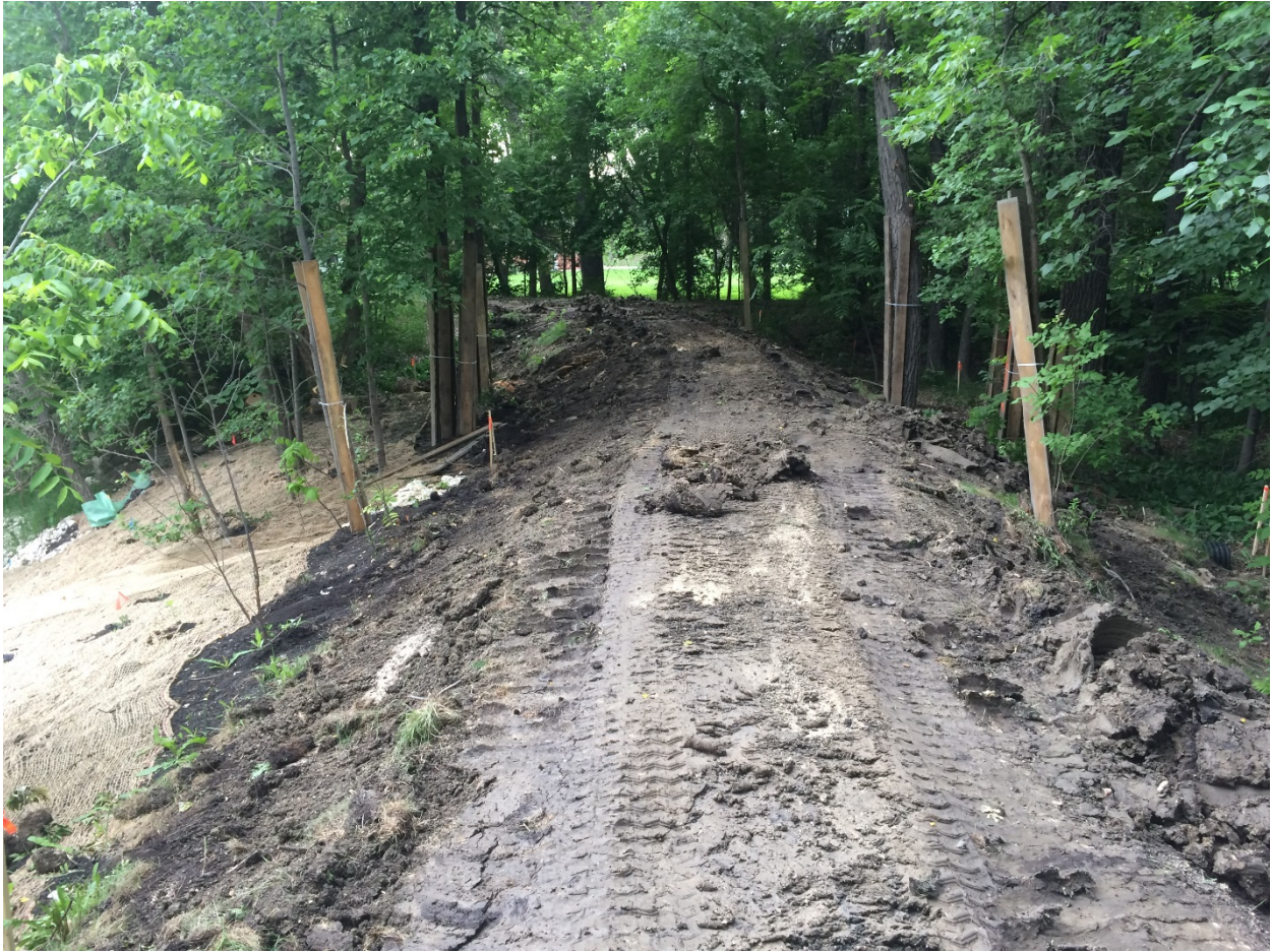
Photo 5 - Existing dike following the removal of organics at 3154 Henderson Highway.
