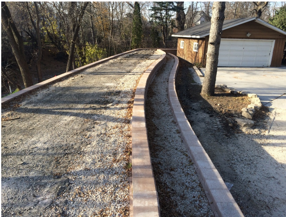
Photo 14 - Dike at 3144 Henderson Highway, prior to topsoil placement.
