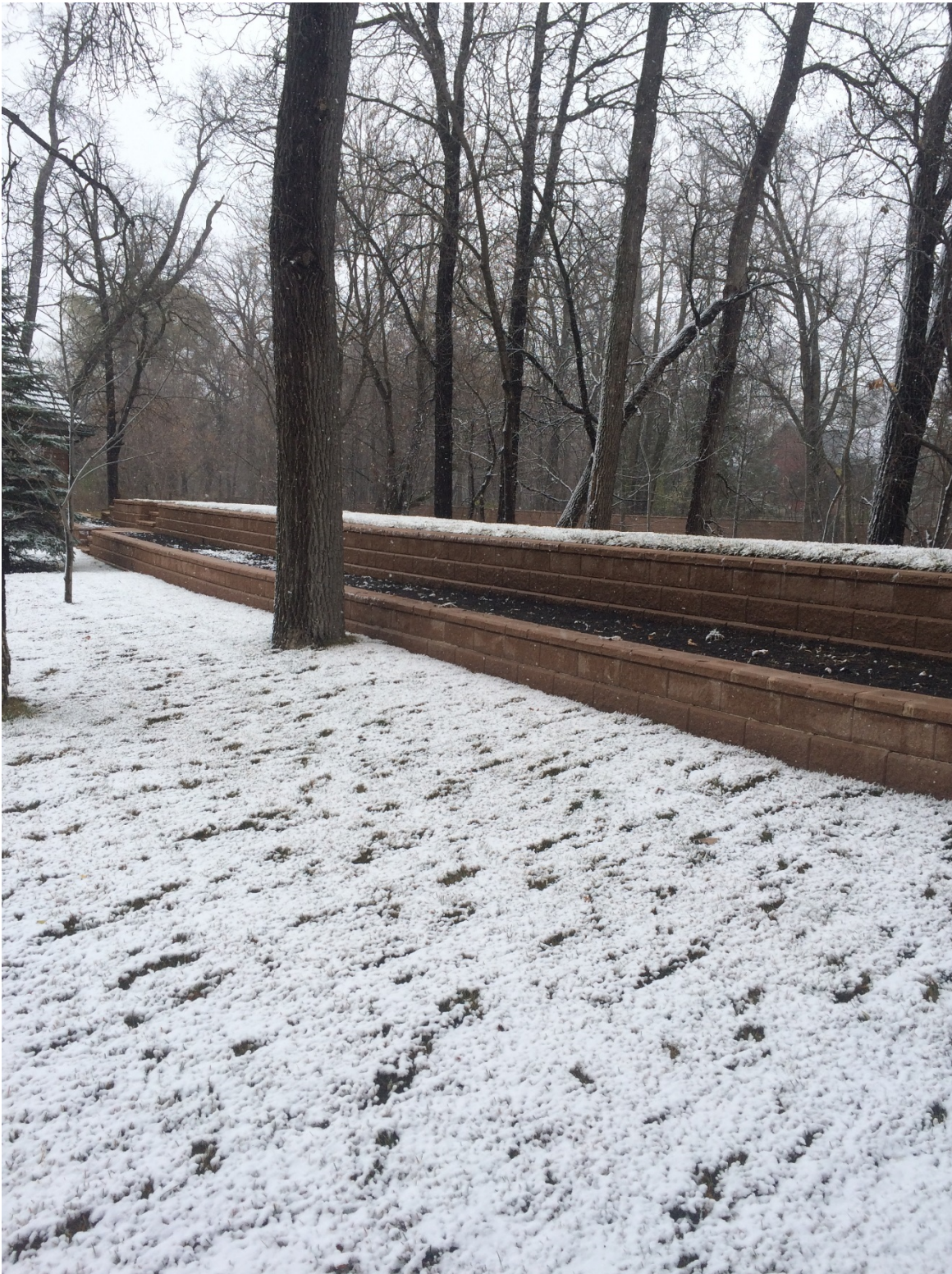
Photo 10 - Dike at 1040 Highland Park Drive.
