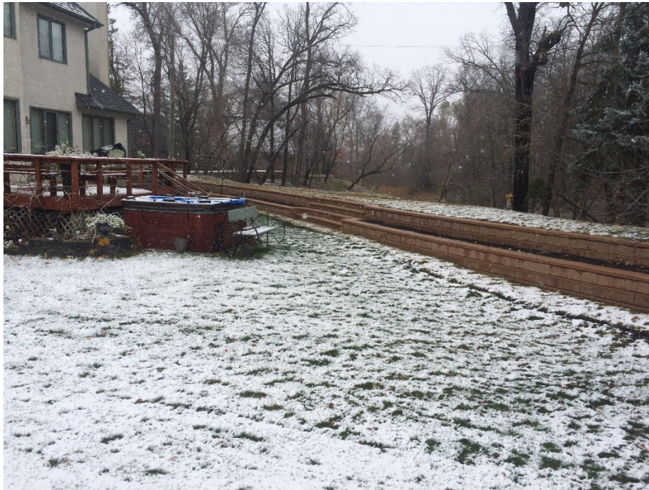
Photo 5 - Dike at 1030 Highland Park Drive.
