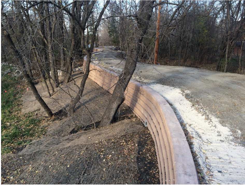
Photo 15 - Dike at 3144/3154 Henderson Highway, prior to topsoil placement.
