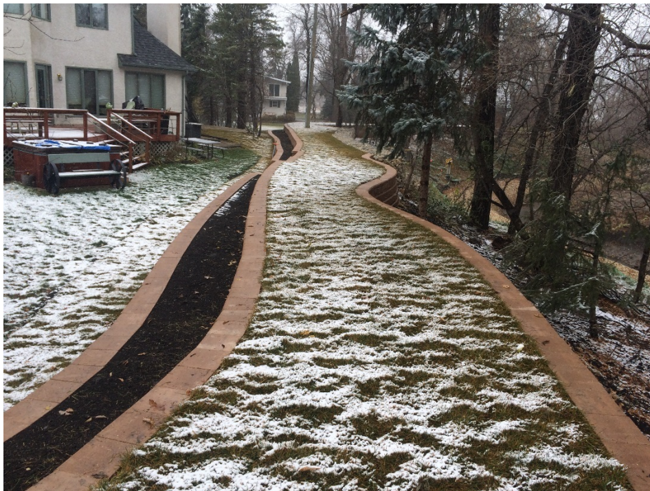
Photo 6 - Dike at 1030 Highland Park Drive.
