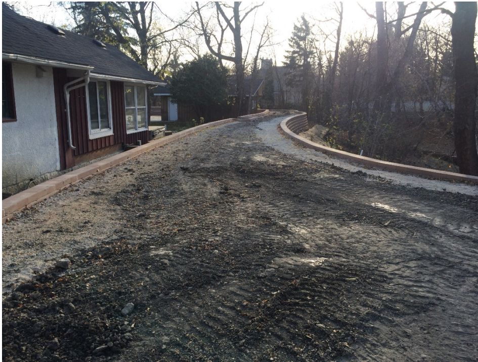
Photo 13 - Dike at 3144 Henderson Highway, prior to topsoil placement.
