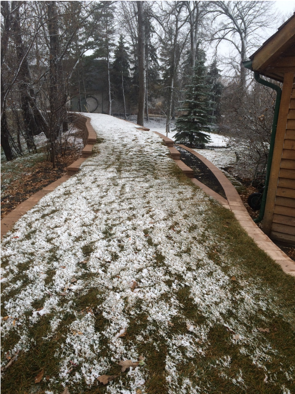
Photo 12 - Dike at 1040 Highland Park Drive.
