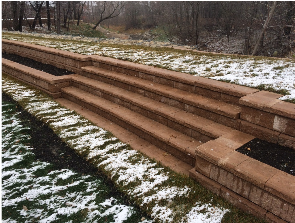
Photo 7 - Stairs at 1030 Highland Park Drive.
