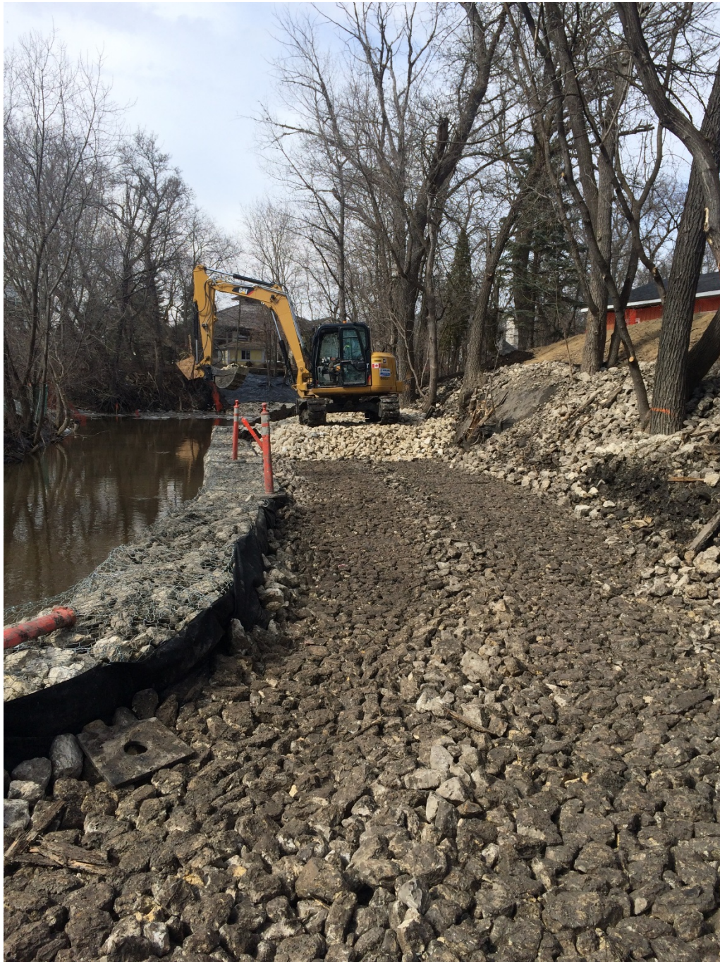
Photo 3 - Placing rockfill toe berm at 3144 Henderson Highway.
