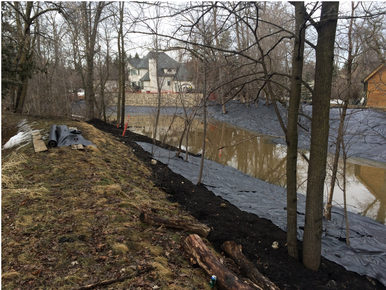
Photo 1 - Topsoil placed with geotextile being placed on top at 3154 Henderson Highway.
