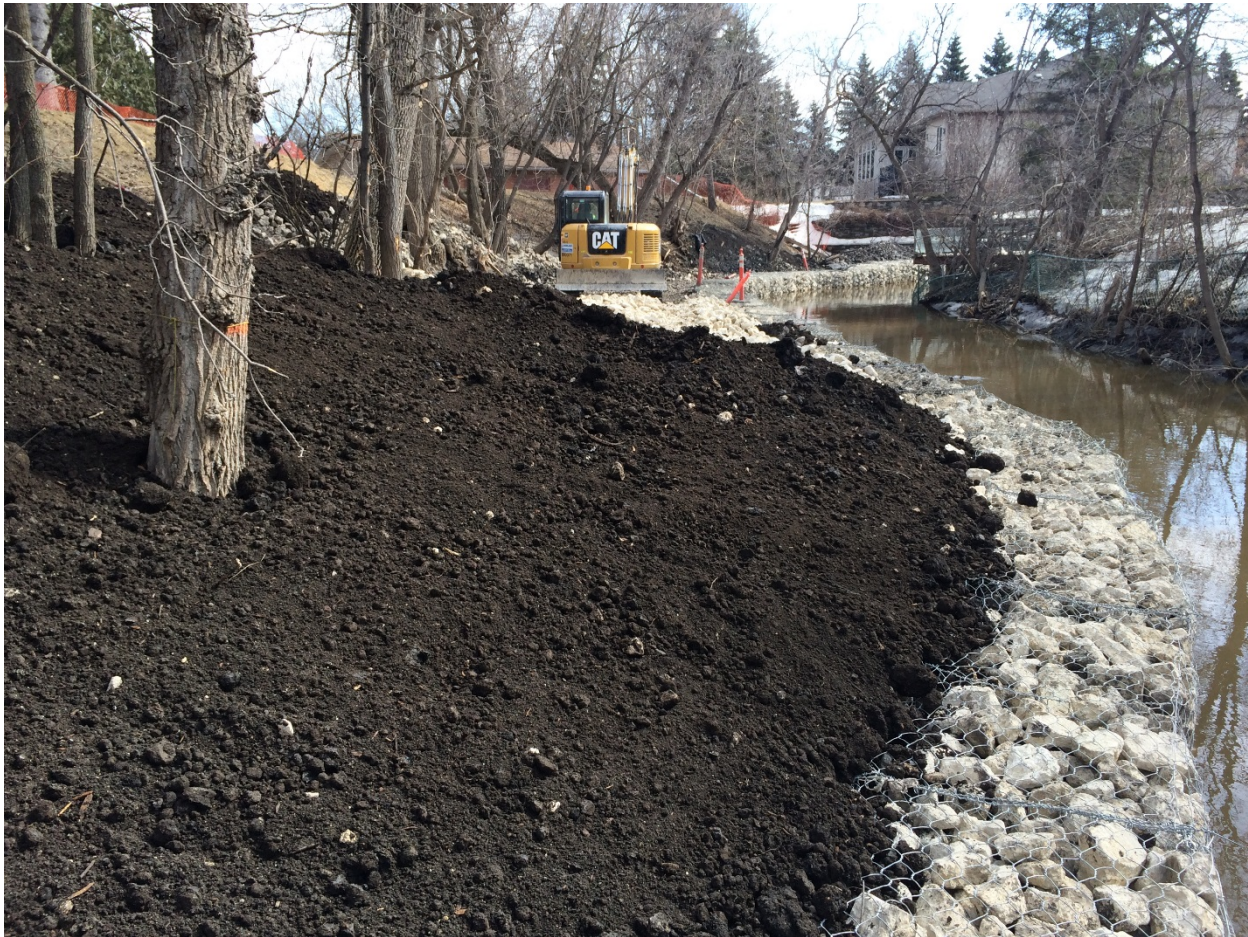
Photo 4 - Placing topsoil on rockfill toe berm at 3144 Henderson Highway.
