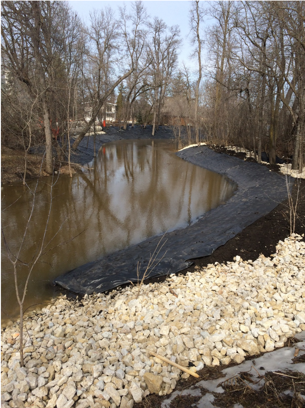
Photo 2 - Topsoil placed with geotextile on top at 3144 Henderson Highway.
