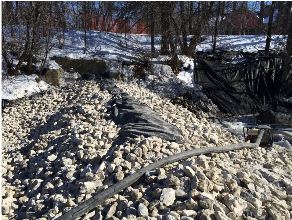
Photo 3 - Pumping water over cofferdam.
