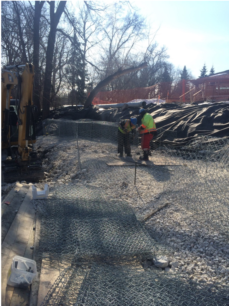
Photo 7 - Installation of gabion baskets at 1030 Highland Park Drive.
