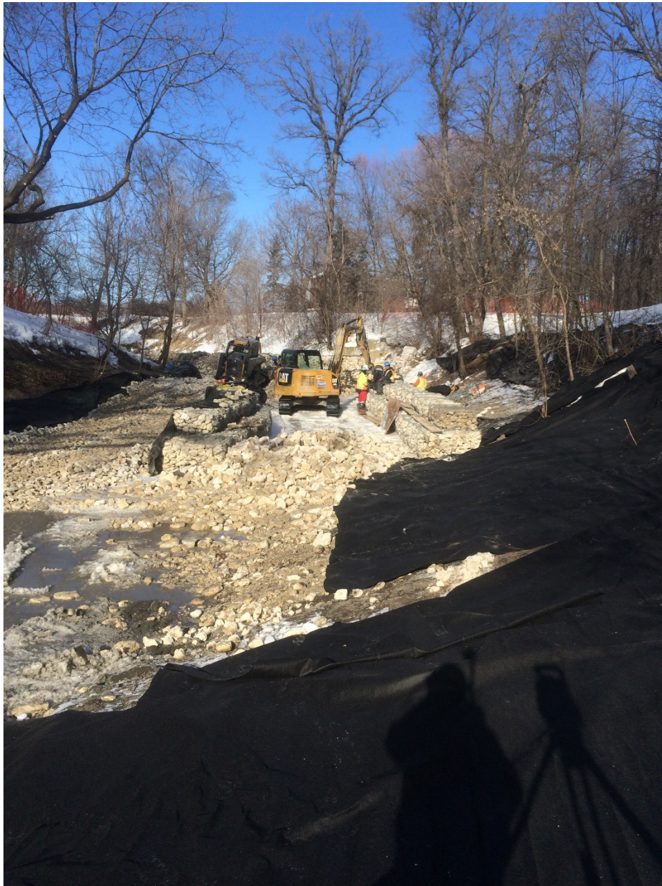
Photo 4 - Completing gabion baskets at 1040 Highland Park Drive and 3154 Henderson Highway.
