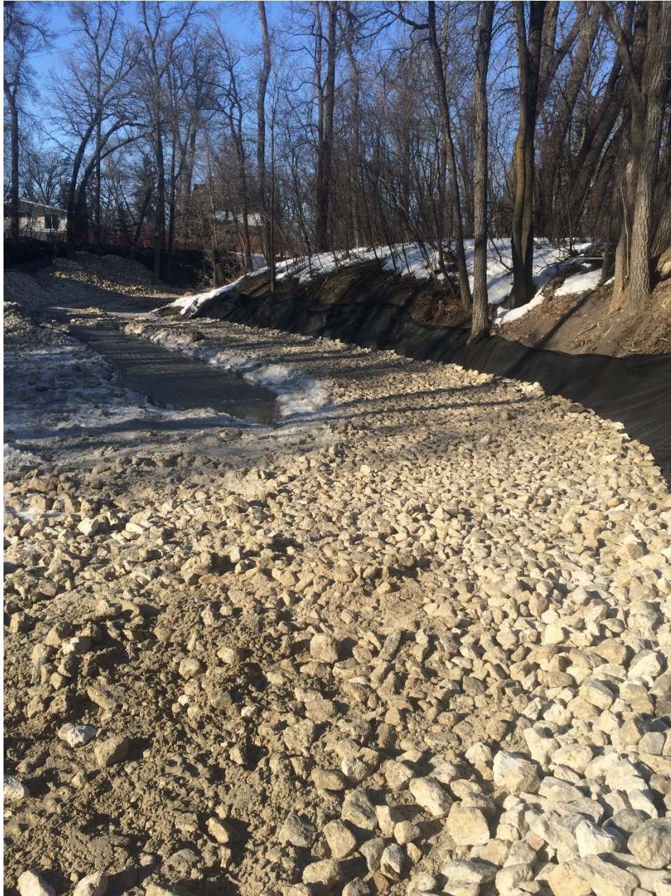
Photo 6 - Rockfill toe berm placement at 3144 Henderson Highway.
