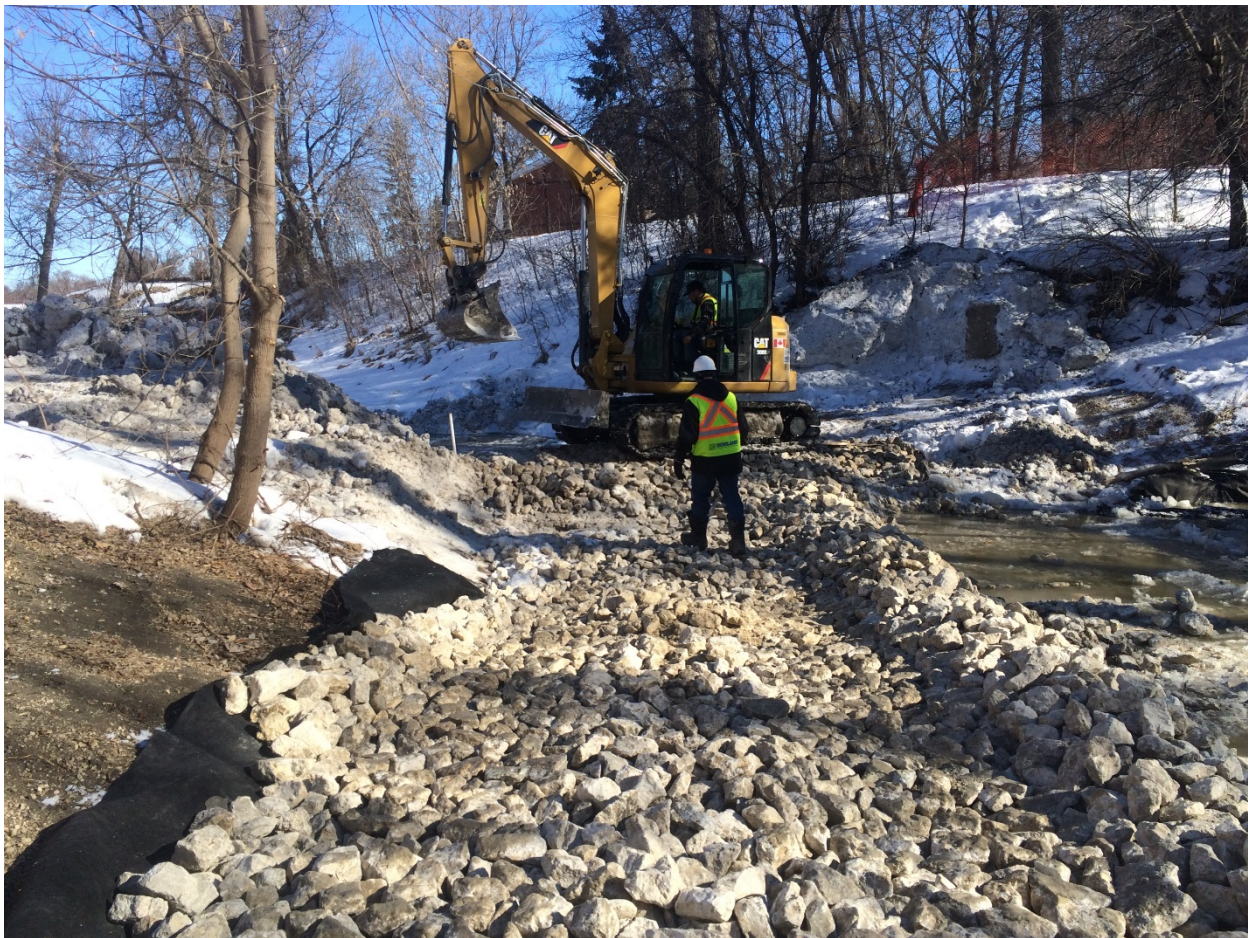
Photo 1 - Cofferdam construction at downstream end of the site.
