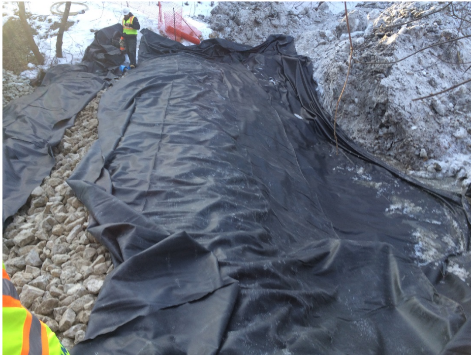
Photo 2 - Liner installation on the cofferdam.
