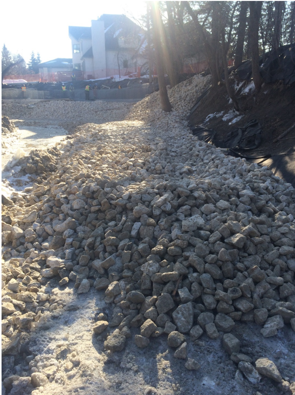
Photo 5 - Rockfill toe berm placement at 1040 Highland Park Drive.
