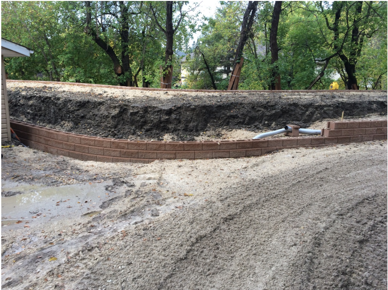
Photo 8 - House side segmental block wall placement at 3144 Henderson Highway.
