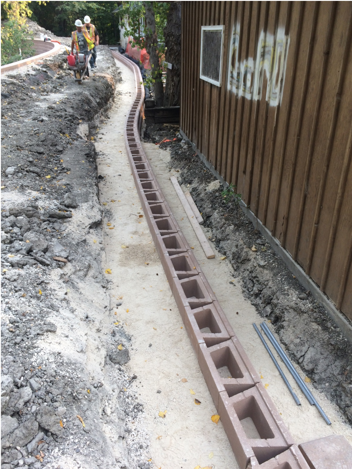
Photo 2 - House side segmental block wall placement at 3144 Henderson Highway.
