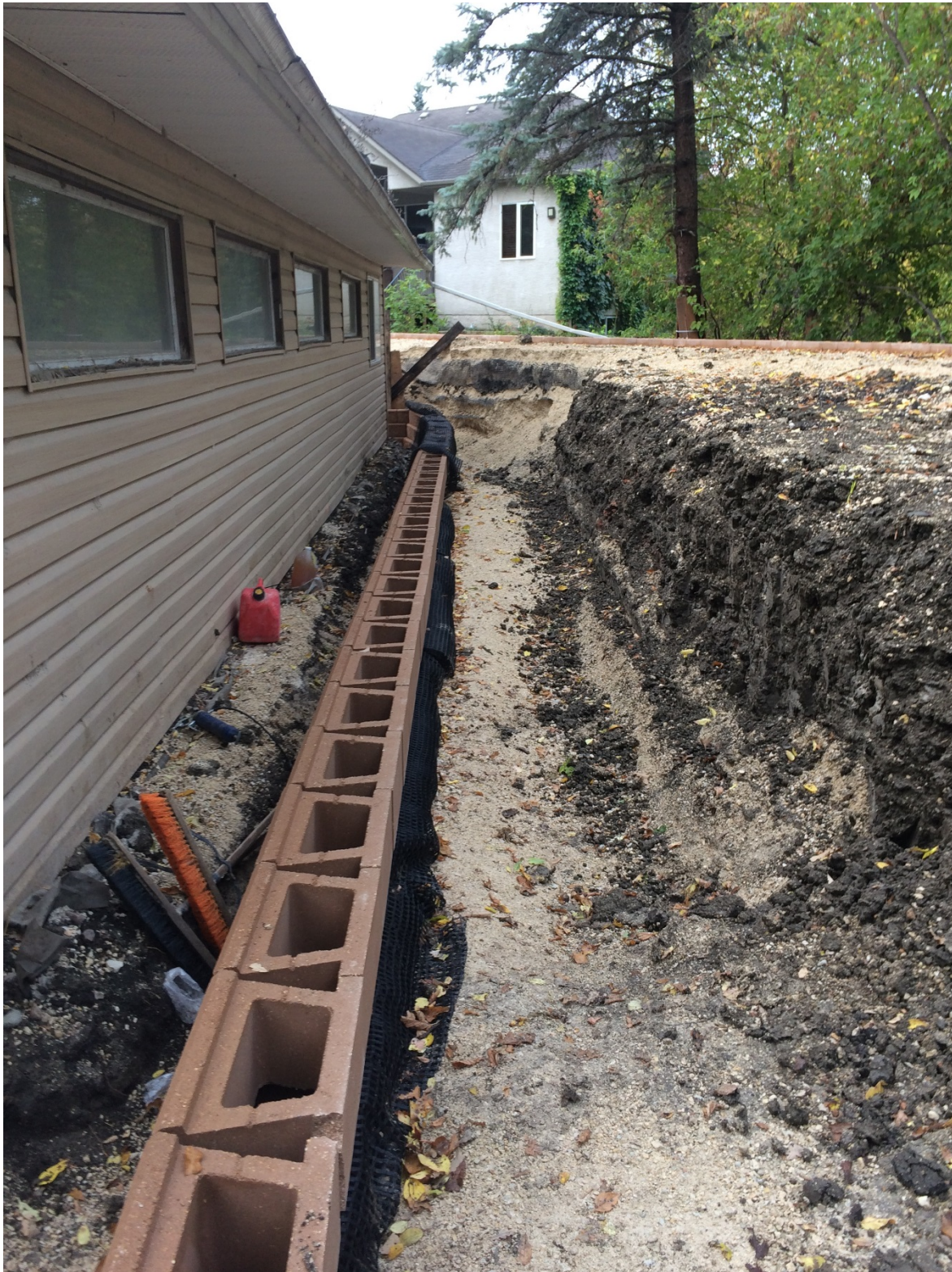
Photo 7 - House side segmental block wall placement at 3144 Henderson Highway.
