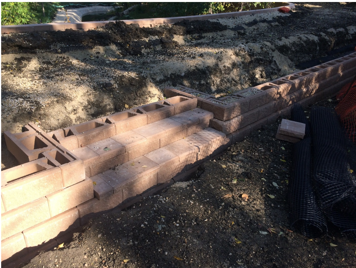
Photo 1 - Stair construction at 3144 Henderson Highway.
