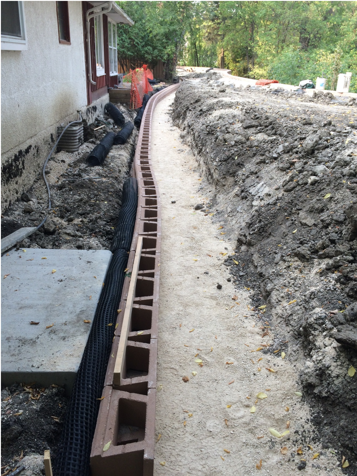
Photo 3 - House side segmental block wall placement at 3144 Henderson Highway.
