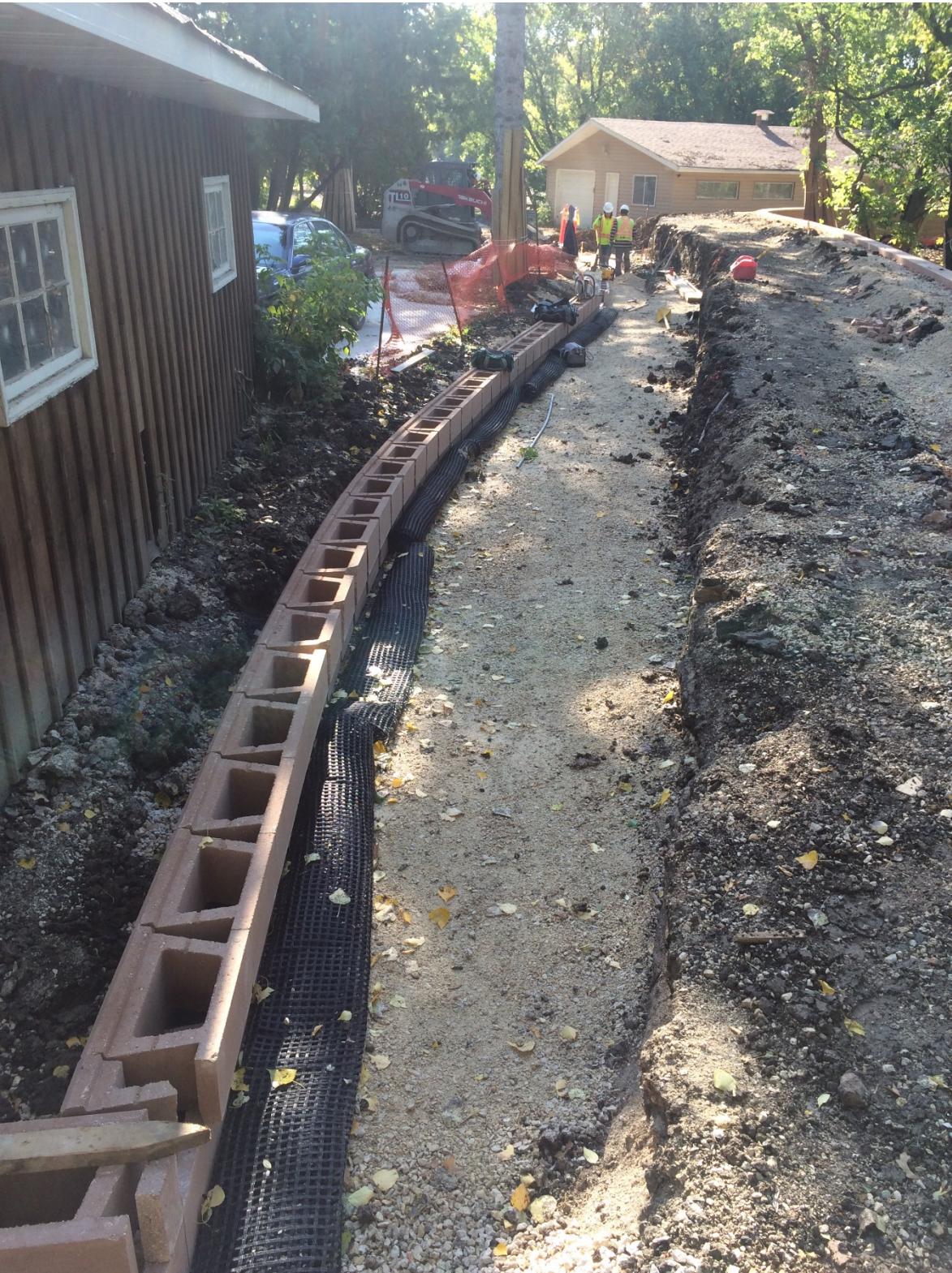
Photo 4 - House side segmental block wall placement at 3144 Henderson Highway.
