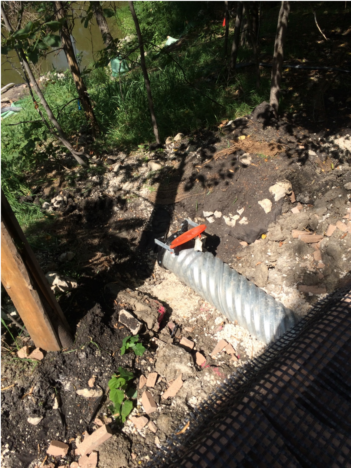
Photo 25 - Flap gate placed on culvert at 3144 Henderson Highway.
