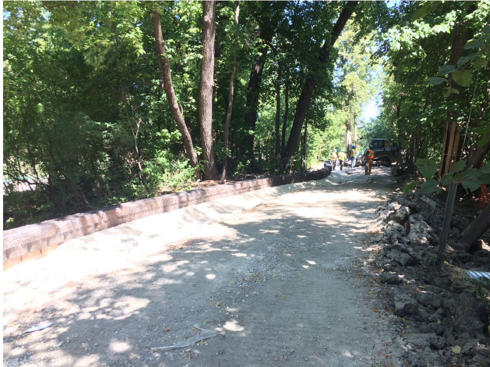
Photo 11 - Placement of the creek side segmental block wall at 3154 Henderson Highway.
