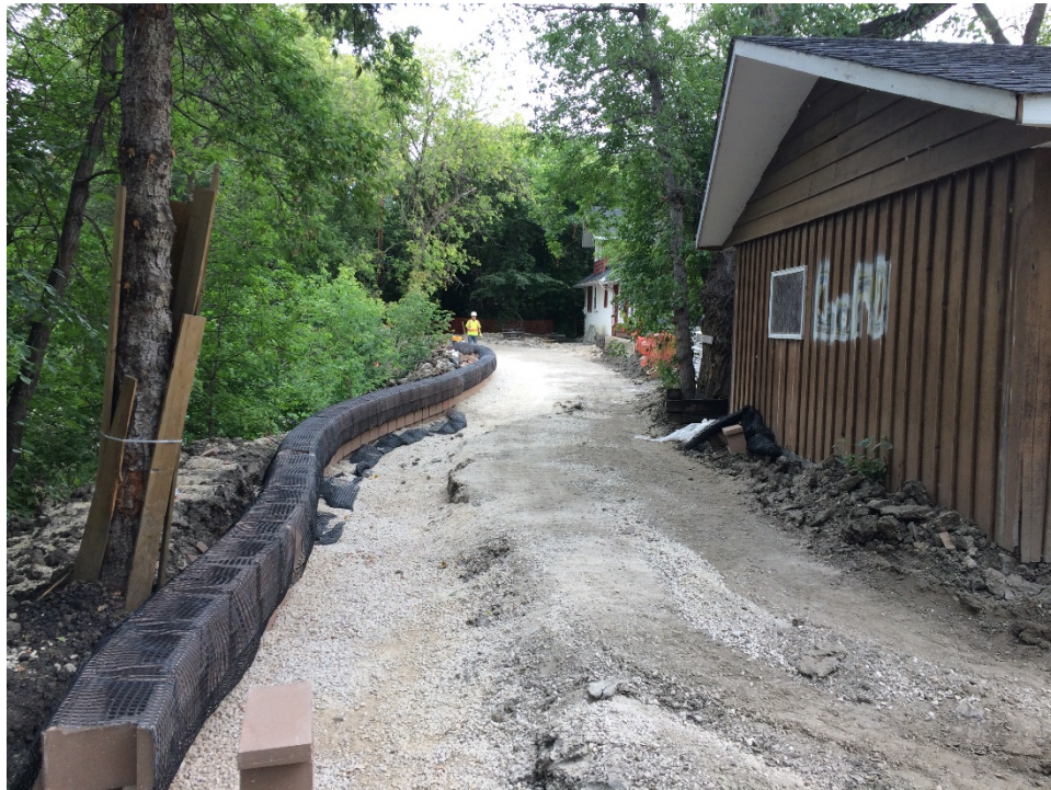
Photo 9 - Placement of the creek side segmental block wall at 3144 Henderson Highway.
