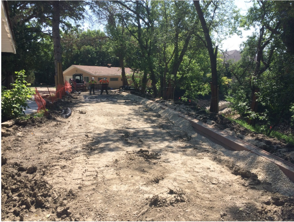
Photo 7 - Segmental block wall placement at 3144 Henderson Highway.
