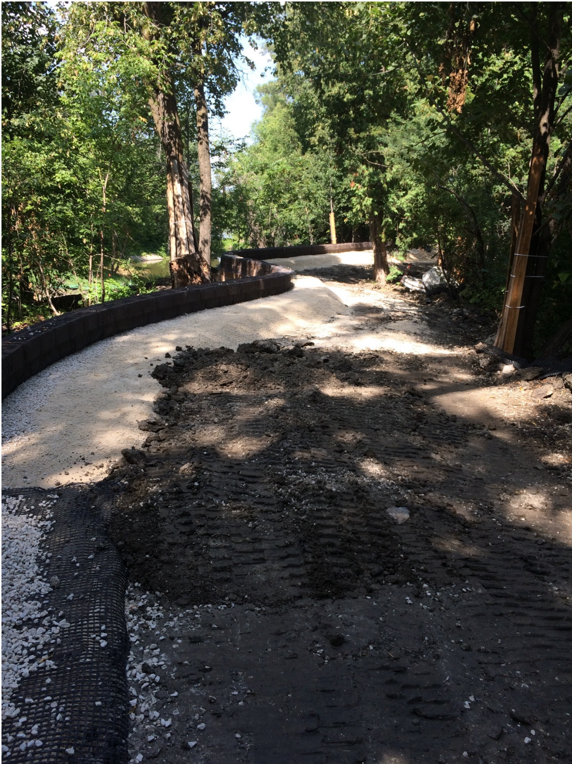
Photo 22 - Final height of creek side segmental block wall at 3154 Henderson Highway.
