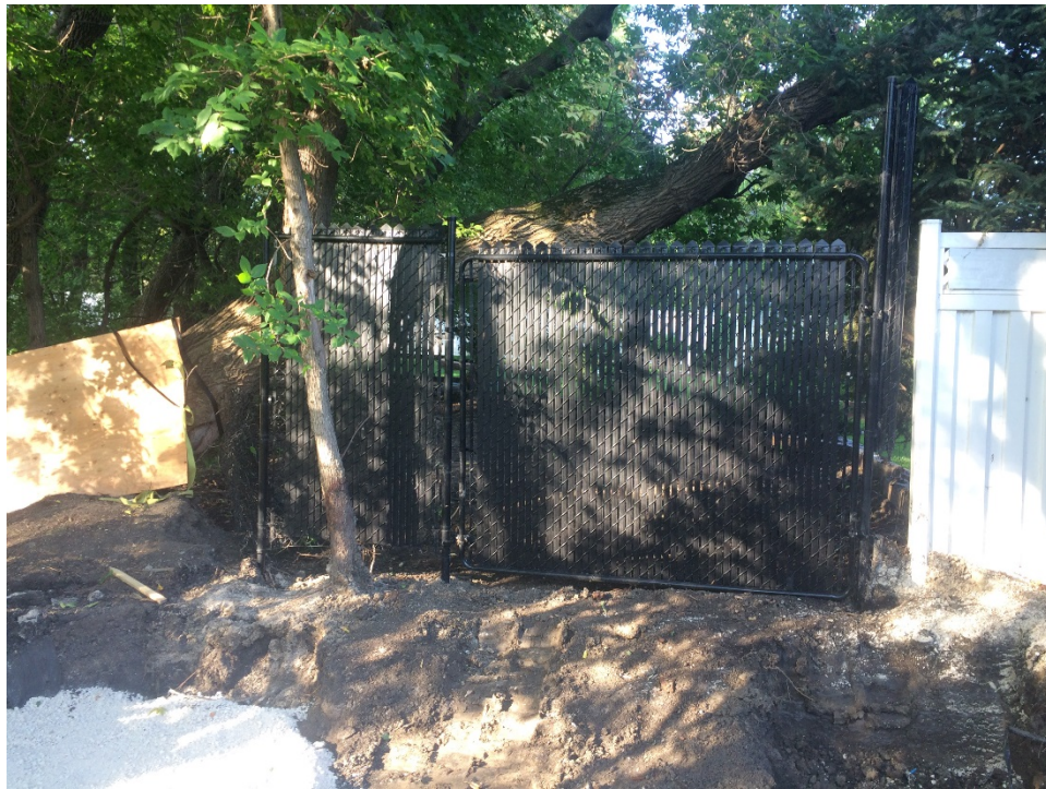
Photo 4 - Fence replaced at new ground elevation between 1010 and 1020 Highland Park Drive.
