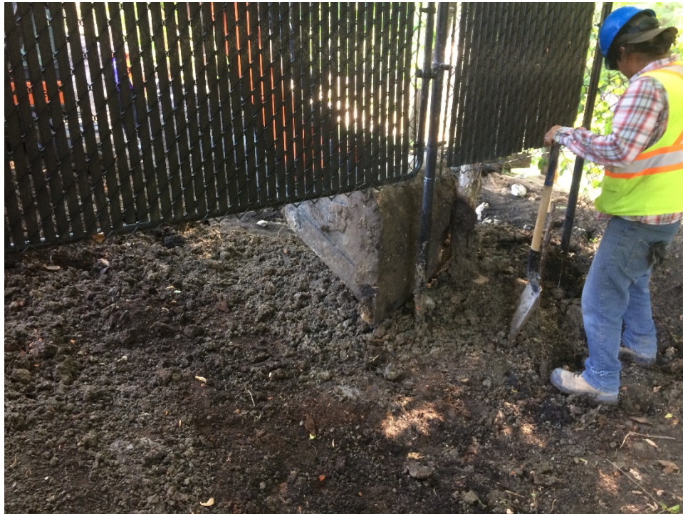
Photo 3 - Removal of existing dike below fence between 1010 and 1020 Highland Park Drive.
