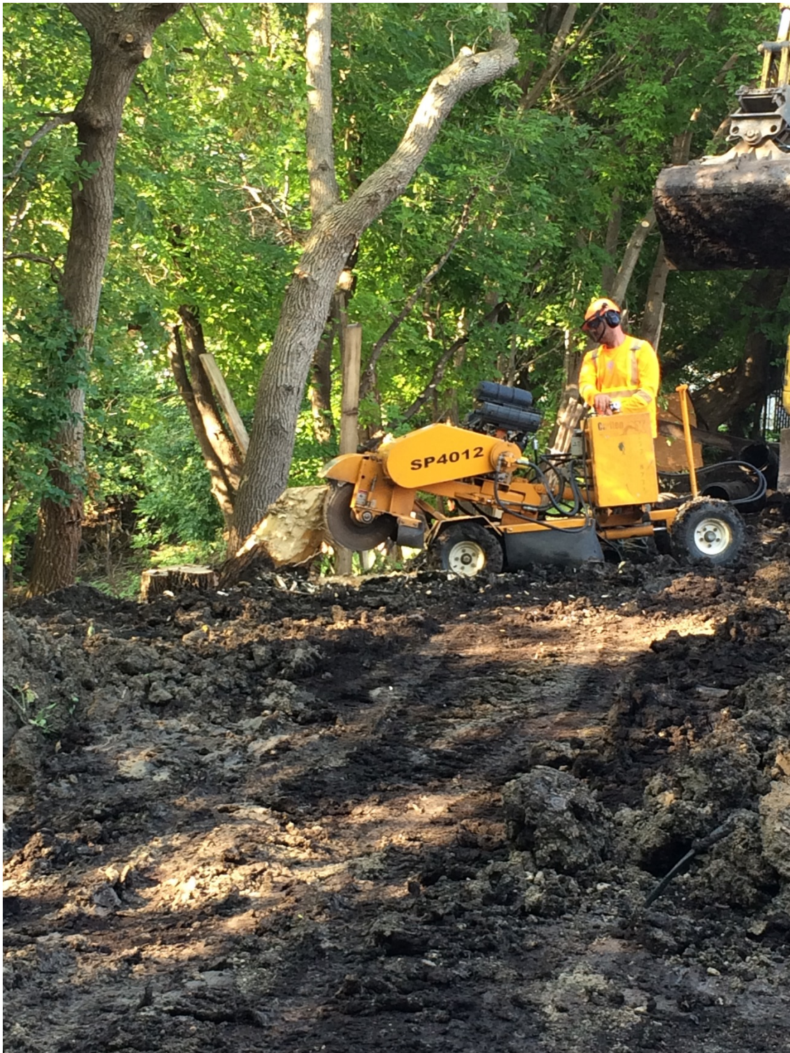
Photo 1 - Arborists removing stumps at 1020 Highland Park Drive.
