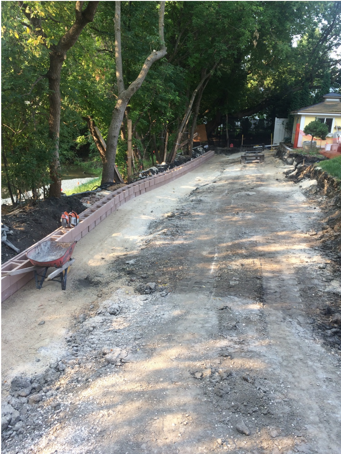
Photo 18 - Segmental block wall placement at 1020 Highland Park Drive.
