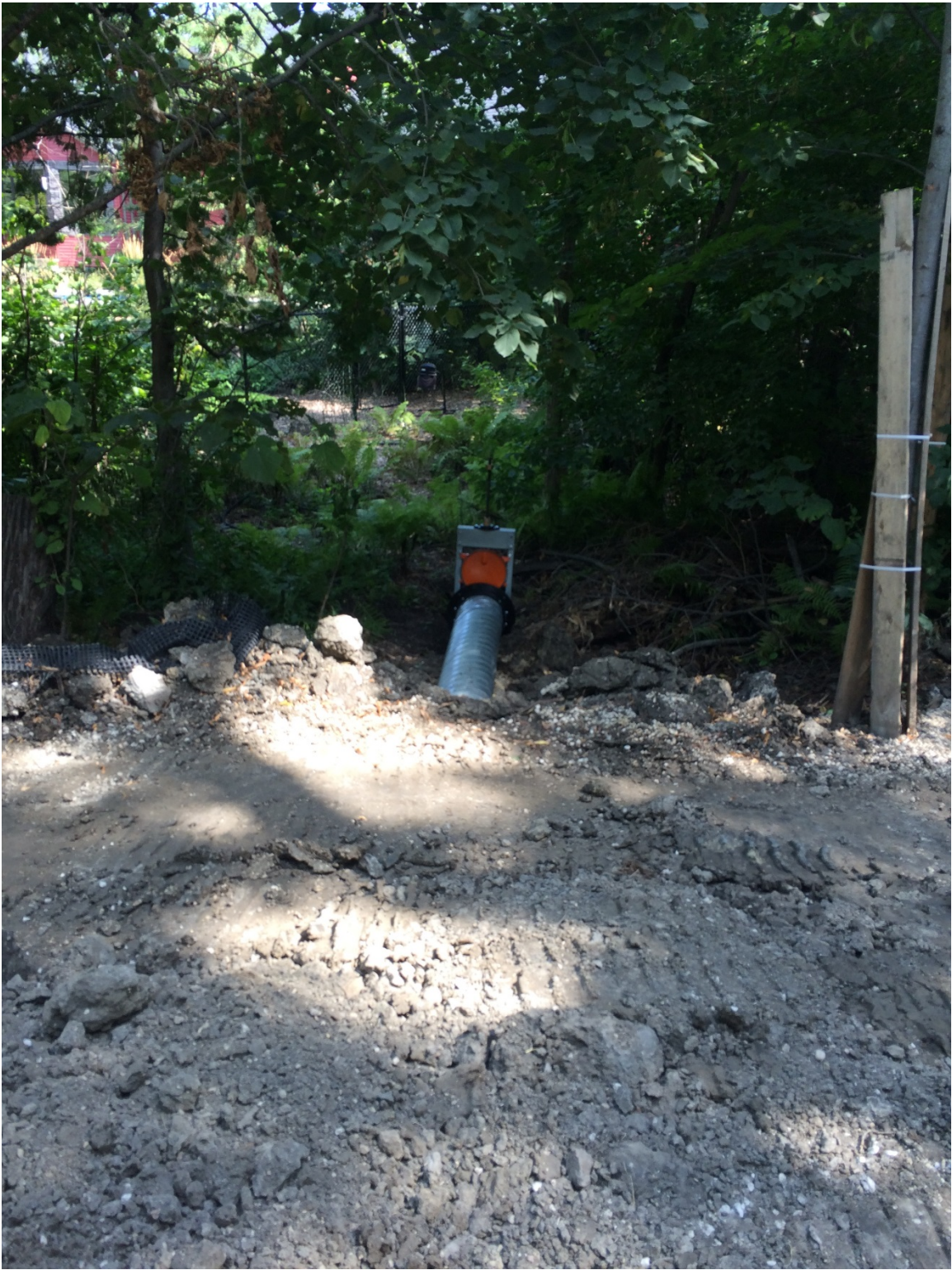
Photo 24 - Canal gate placed on culvert at 3154 Henderson Highway.
