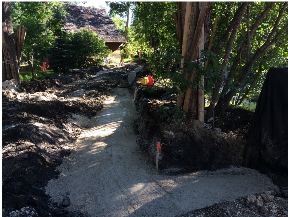
Photo 12 - Foundation of creek side segmental block wall at 1040 Highland Park Drive.
