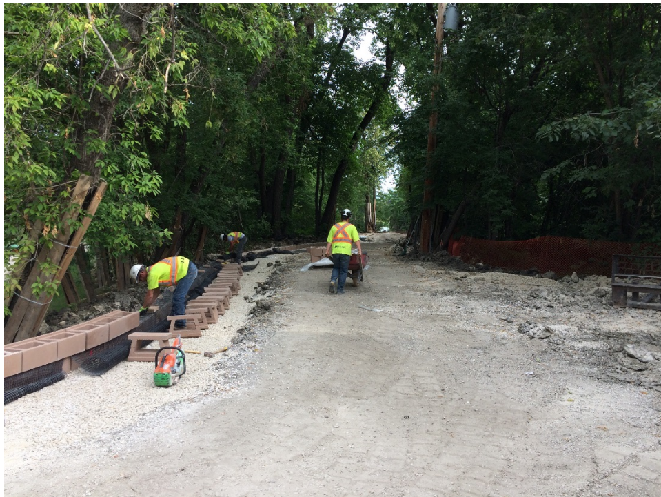
Photo 10 - Placement of the creek side segmental block wall at 3144 Henderson Highway.
